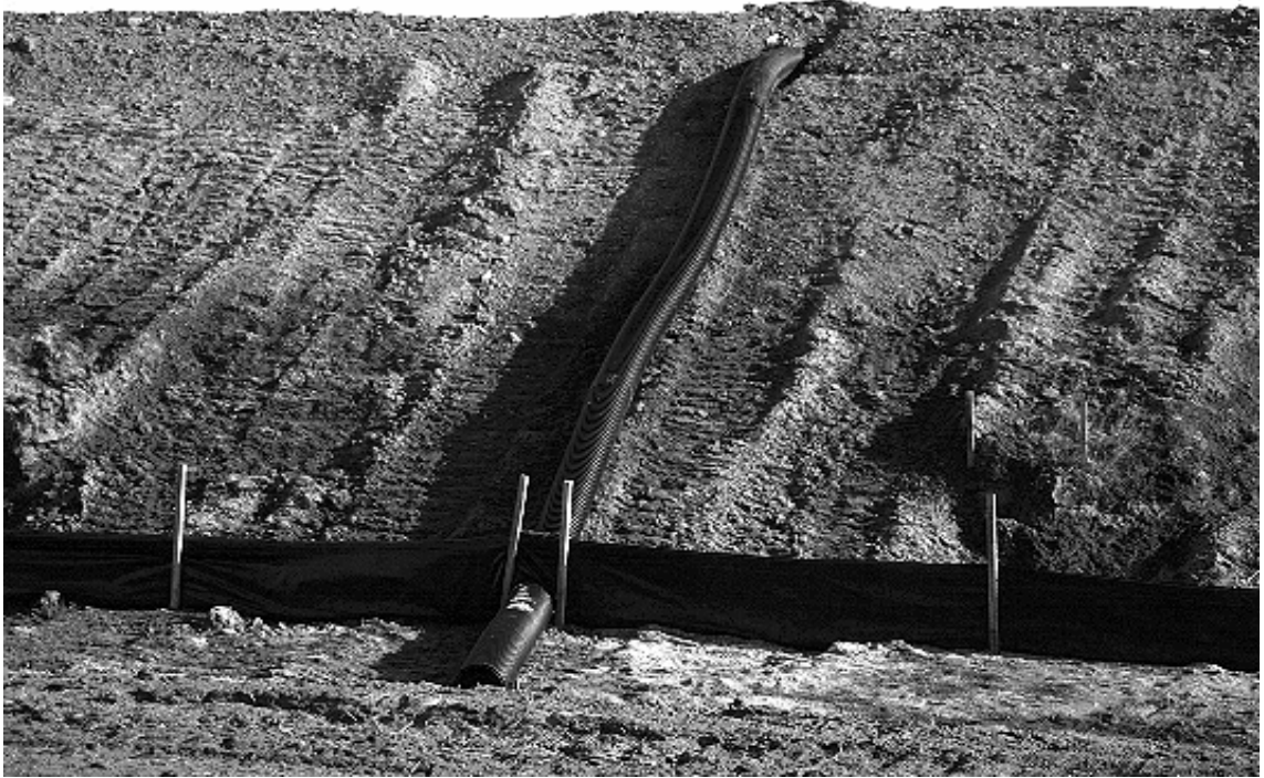
Plate 6: Pipe drop structure
