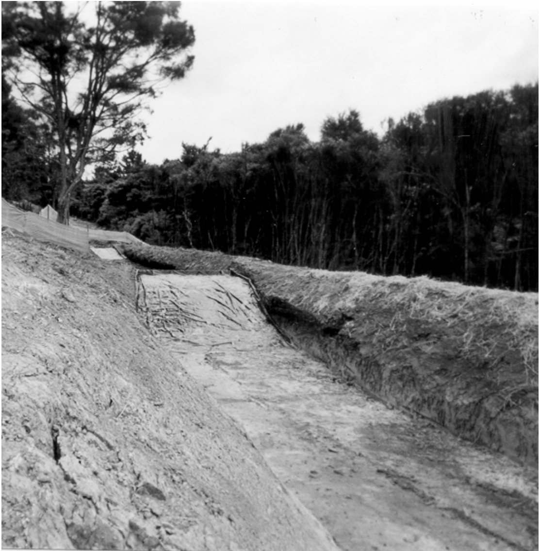
Plate 5: Level spreader with forebay.
