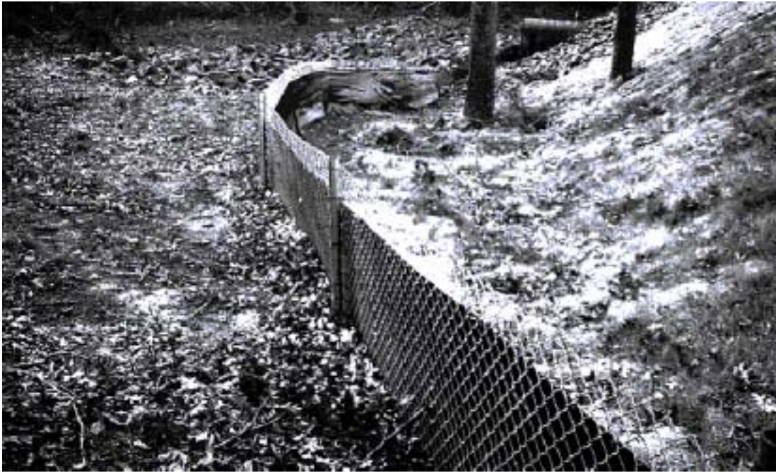
Plate 15: Super Silt Fence
