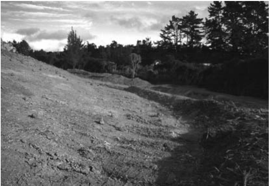
Plate 2: Runoff diversion channel/bund
