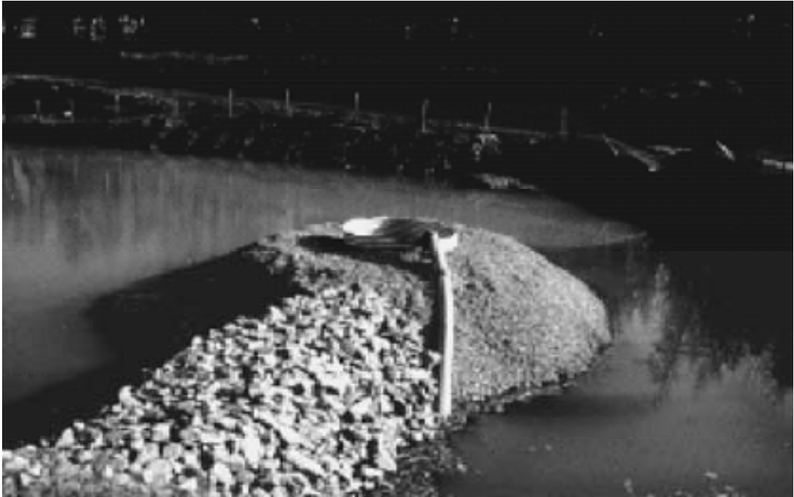
Plate 16: Sump /Sediment Pit
