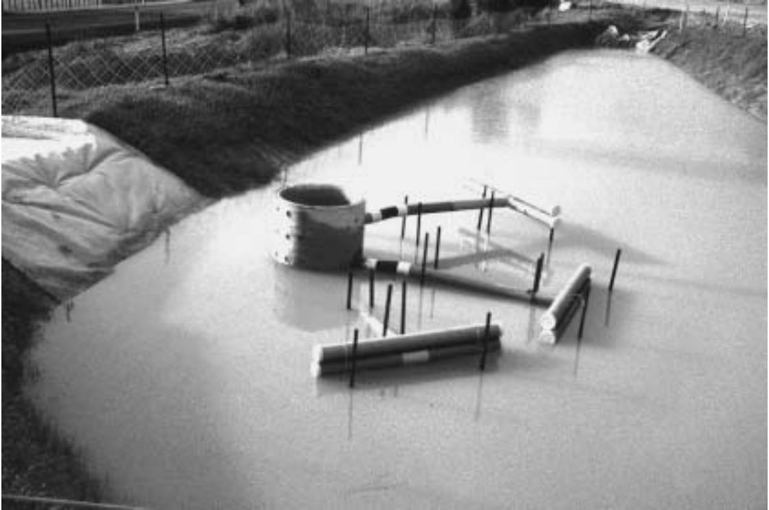
Plate 13: Sediment retention pond showing decant system
