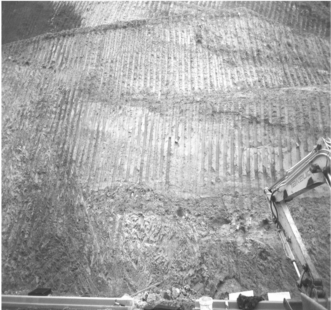
Plate 1: Road cutting showing bedded loess deposit. Fault derived unconformity (bottom left of photograph) separates greywacke parent material from loess, Kaiwharawhara, Wellington.
