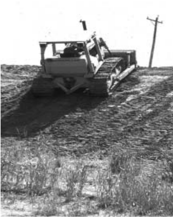
Plate 8: Surface roughening
