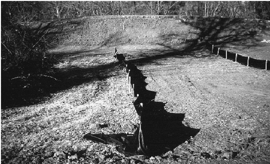
Plate 14: Silt Fence
