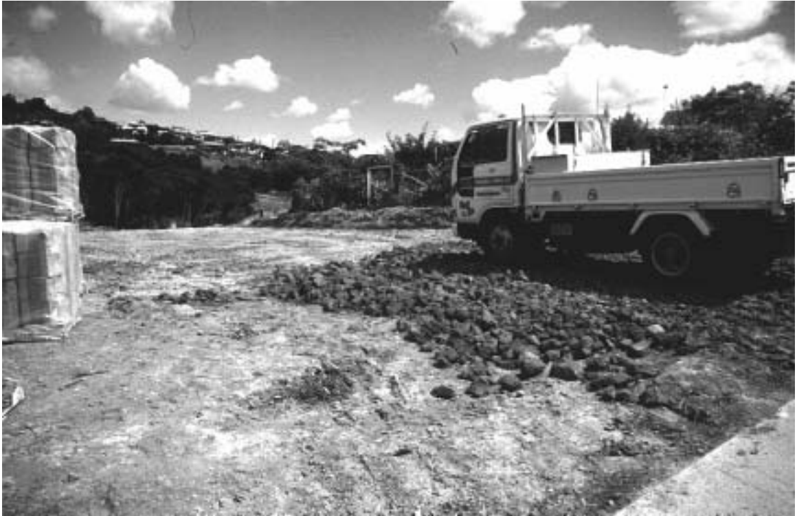
Plate 9: Stabilised construction entrance
