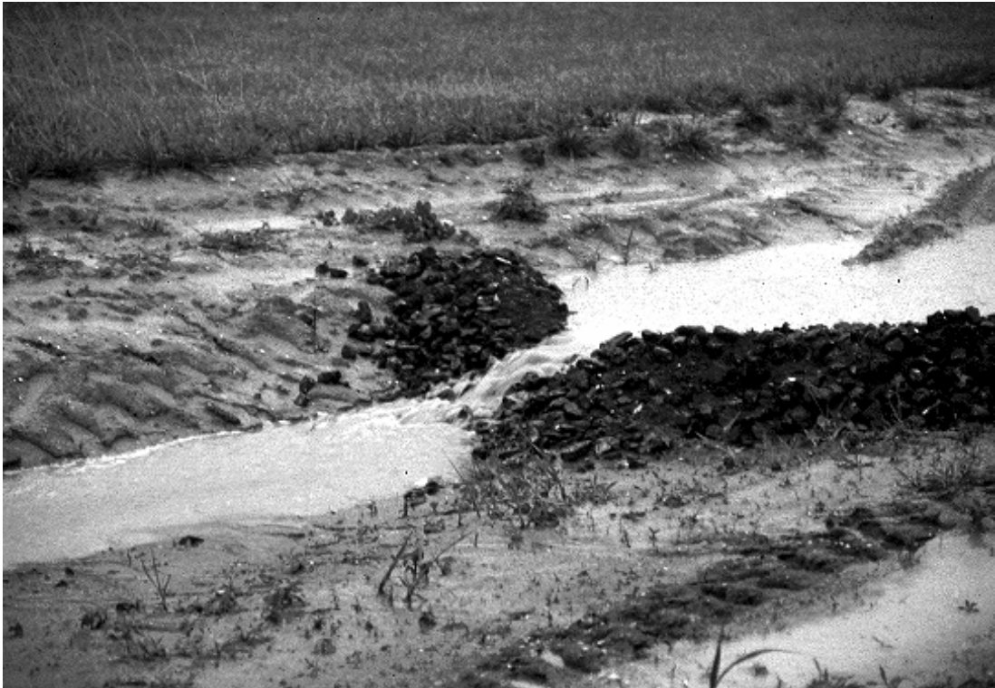
Plate 4: Rock check dam
