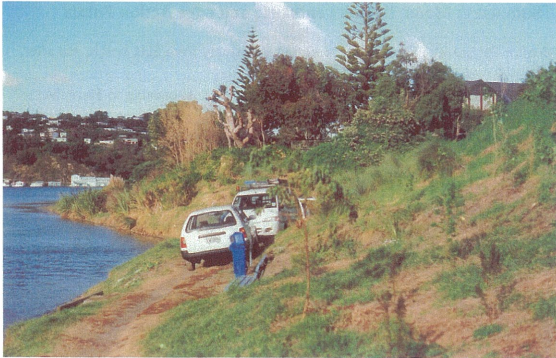
Stabilisation planting between Pascoe Avenue and Camborne Walkway
