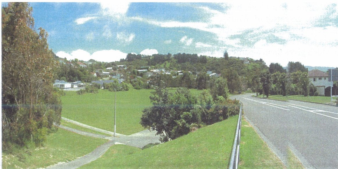
Postgate Drive with hard surfaces and drains.
