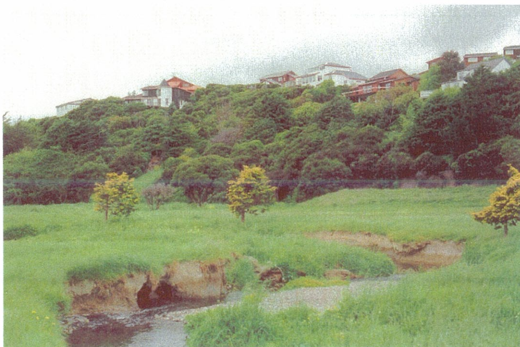
Bank erosion at the bottom end of Duck Creek
