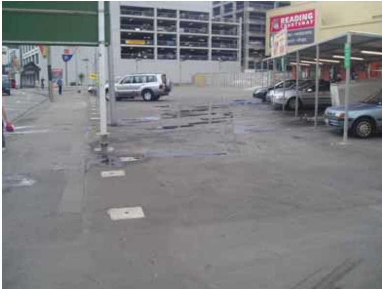
Car grooming water enters the gutter outside Wash'n'shop
