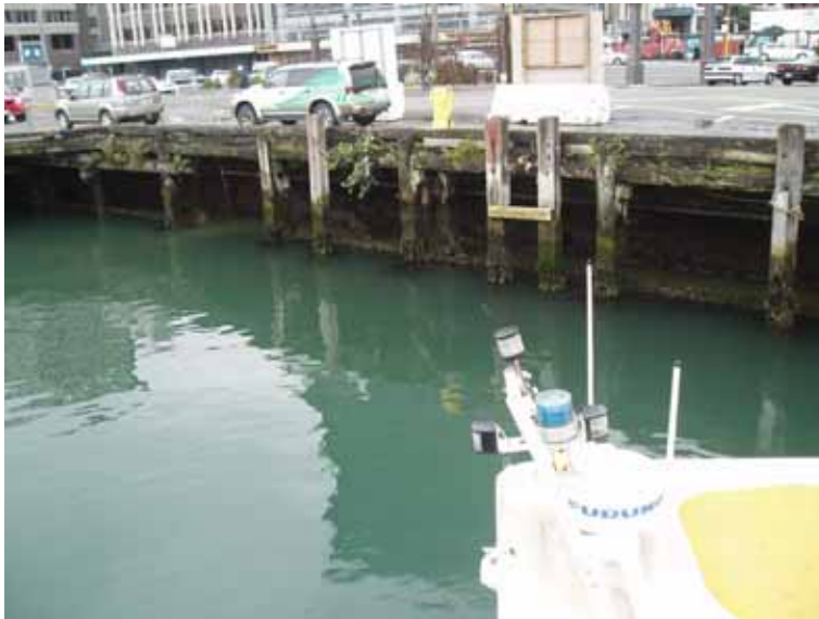
Wellington Harbour where raw sewage was discharged
