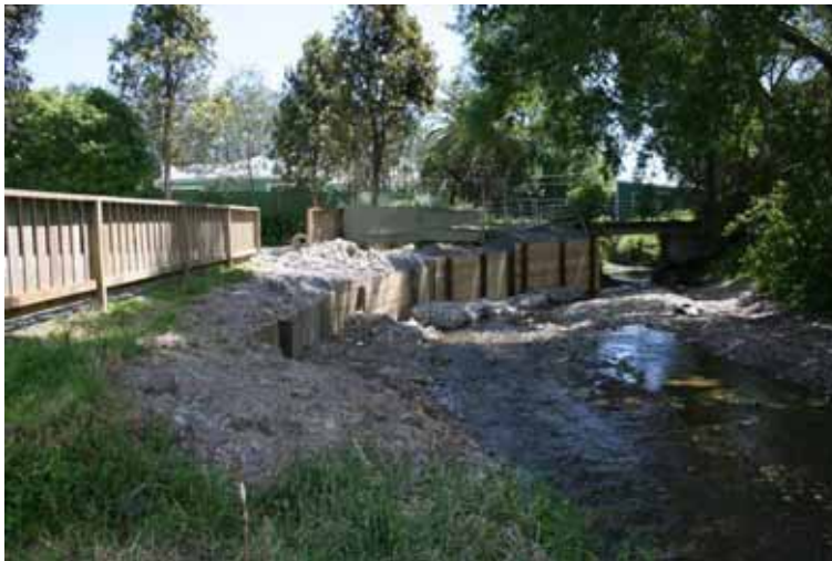
A timber wall in Wharemauku Stream
