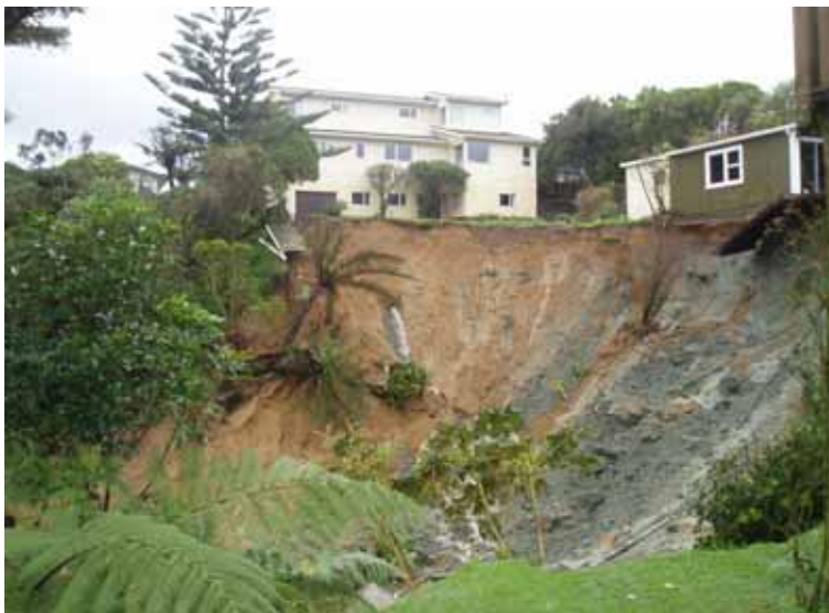
A landslide in Kelson
