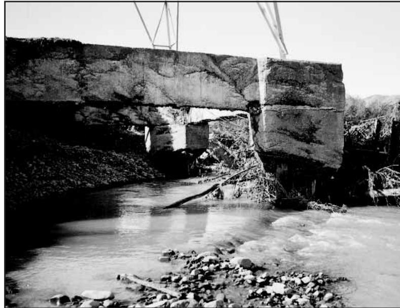
PHOTOGRAPH 7: UNDERMINED LEGS OF THE TRANSPOWER PYLON IN JIM COOK PARK
