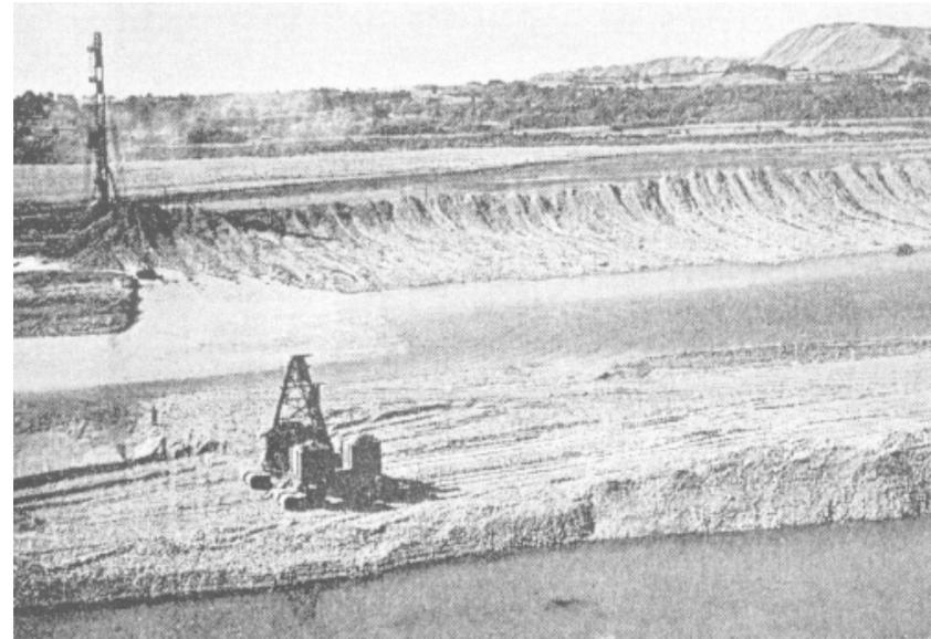
PHOTOGRAPH 11: IN 1946 THE TOWER DREDGE BEGAN A MASSIVE TASK ON THE LOWER OTAKI RIVER (BELOW STATE HIGHWAY 1), EXCAVATING THOUSANDS OF CUBIC METRES OF RIVER GRAVEL THAT NOW CONSTITUTES THE RIGHT STOPBANK THAT PROTECTS OTAKI TOWNSHIP (THE RIVER BED WAS LOWERED BY ABOUT 2 M)
