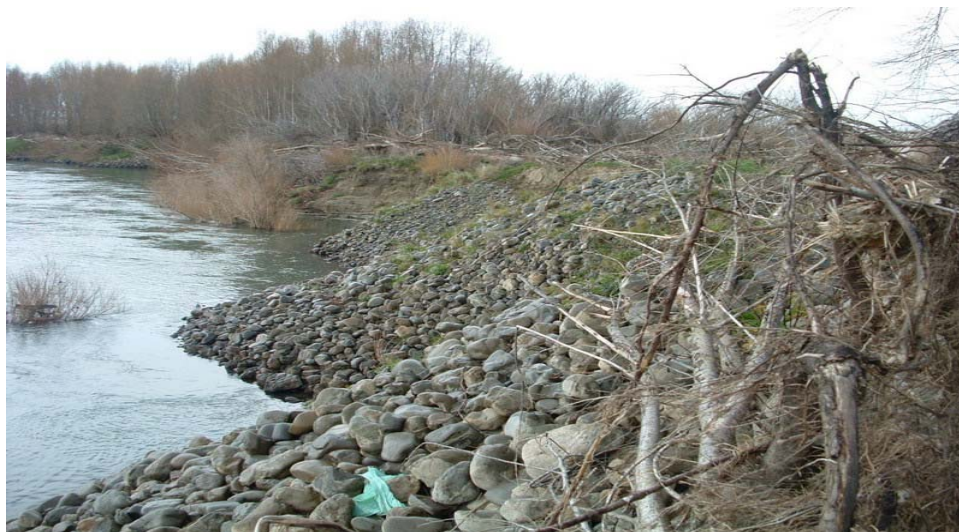
Picture 3: boulder groynes
