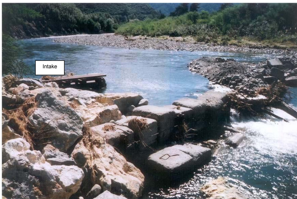
Figure 6 : Longwood Water Race Intake
