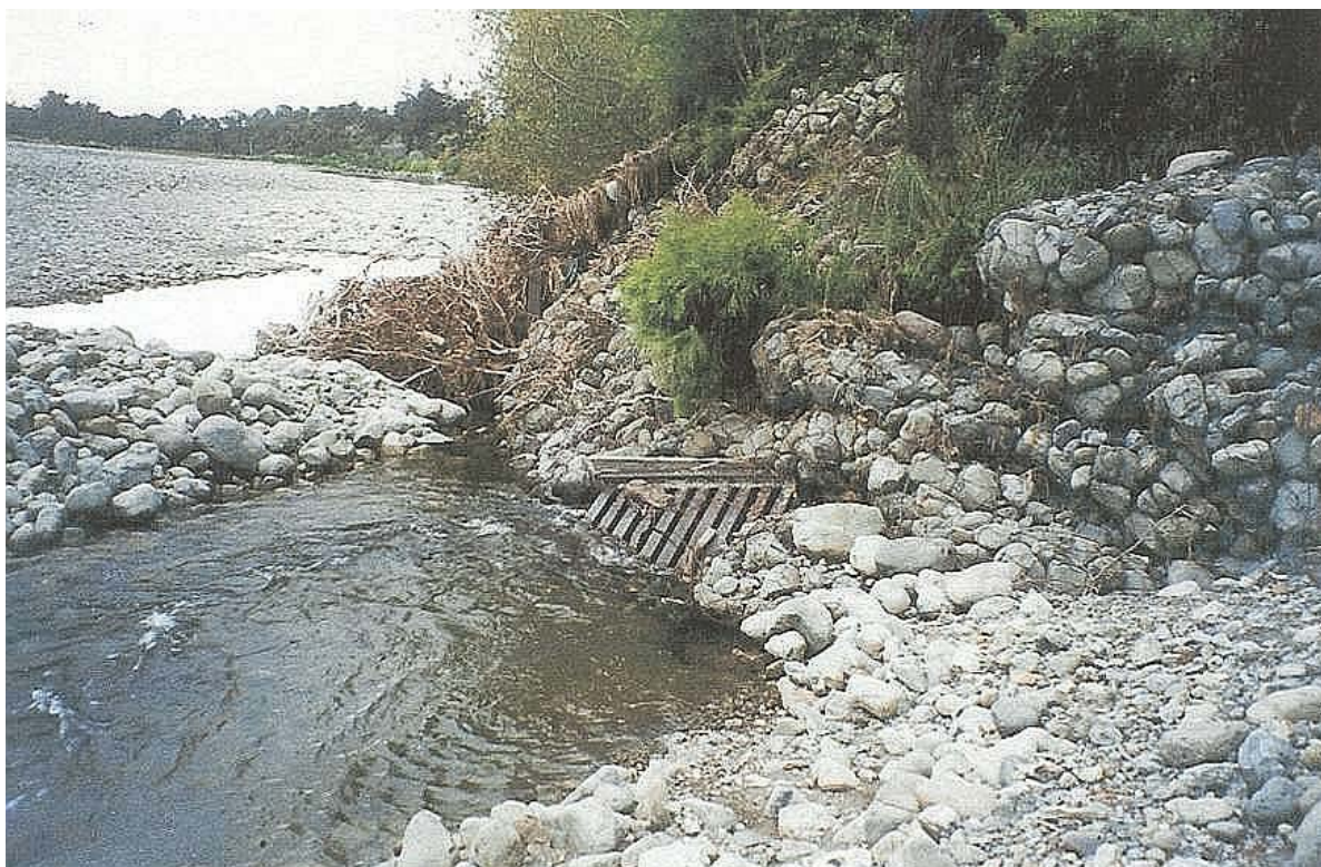
Figure 5 : Moroa Water Race Intake
