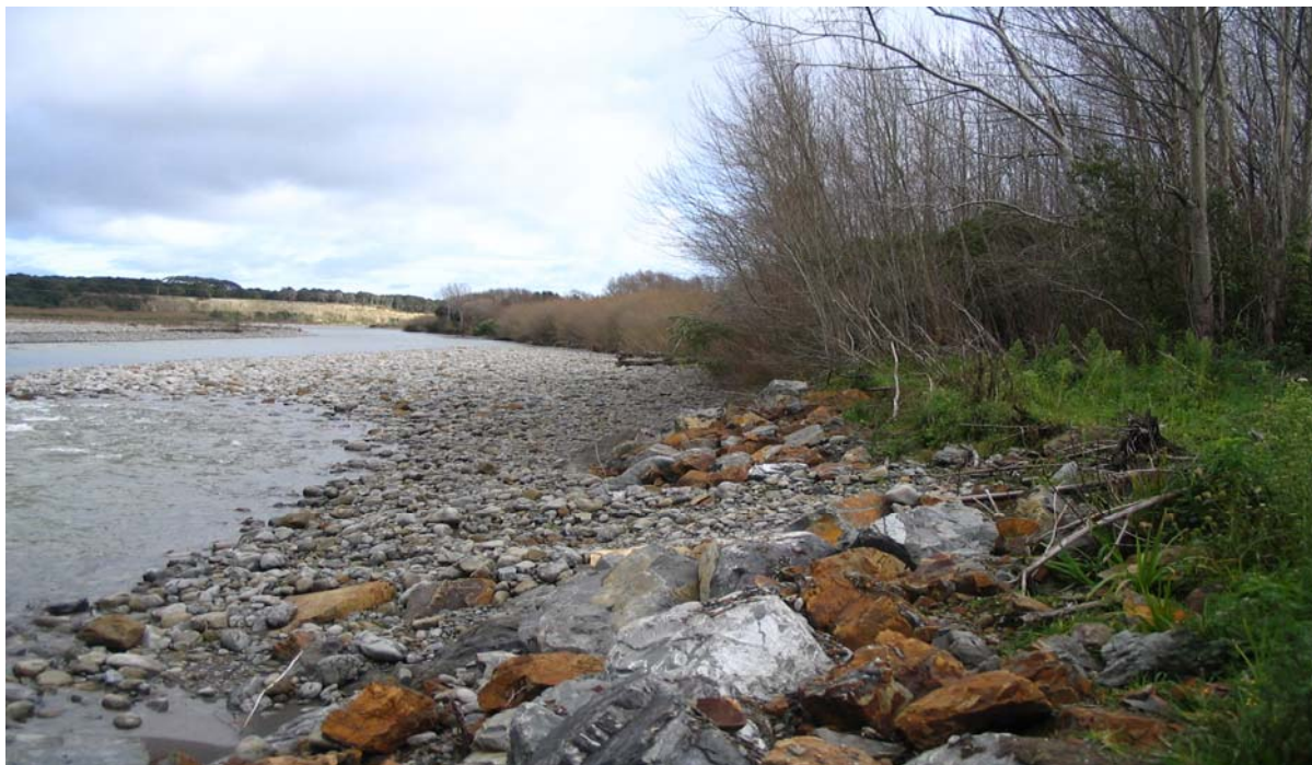
Figure 2 - Upper Taylor’s rockline extension (downstream right bank)
