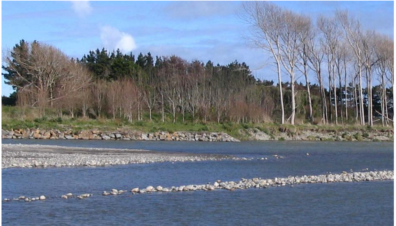
Figure 4 - Leithbridge rockline, left bank. Use of the end groyne to assist in the transition from the rock lining to the unlined bank
