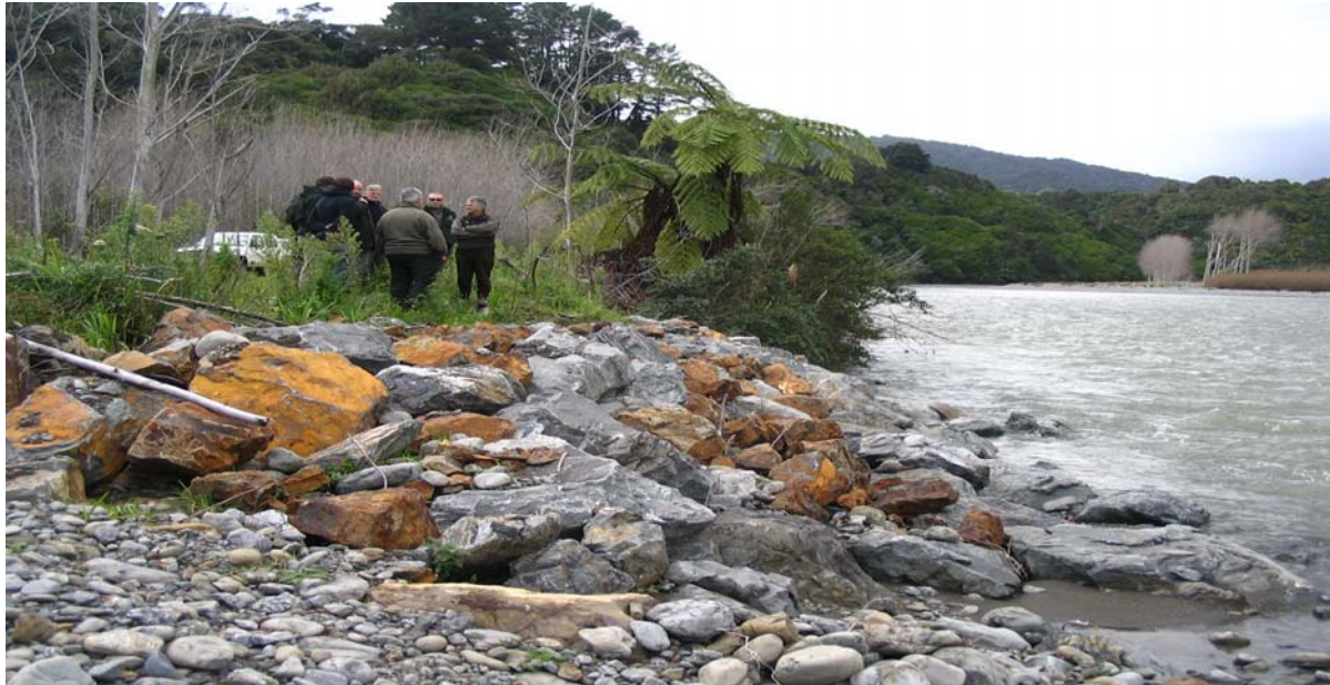
Figure 1 - Upper Taylor’s rockline extension (upstream right bank)
