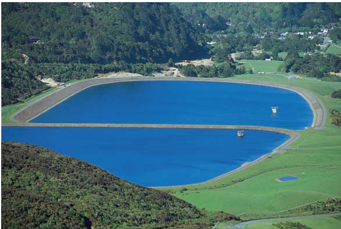
We are preparing to strengthen the Stuart Macaskill Lakes' embankments and upgrade the storage capacity by 13%
