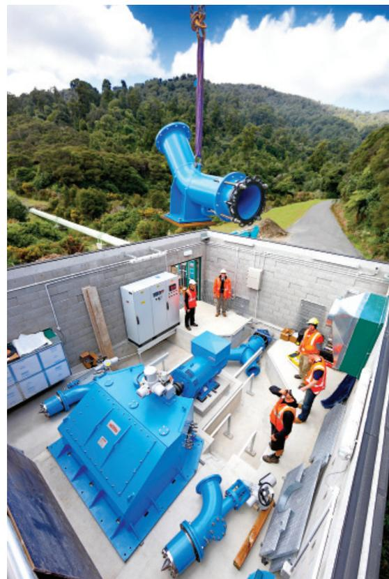
Lowering part of the turbine into the Wainuiomata hydro-electric generator building
