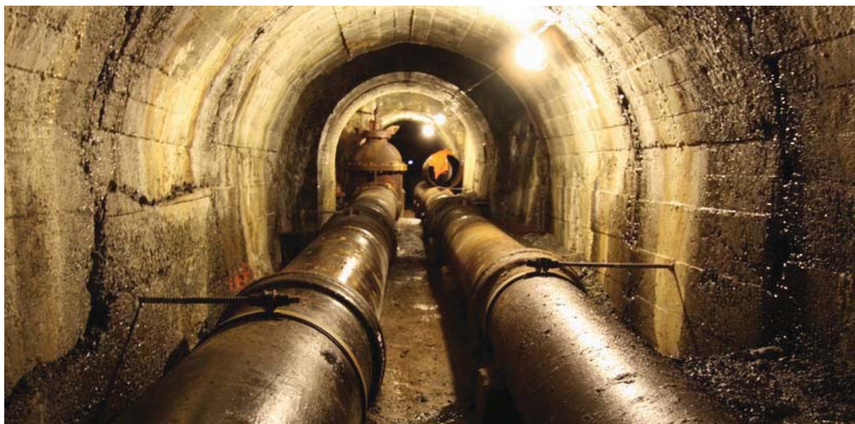
Karori water pipe tunnel
