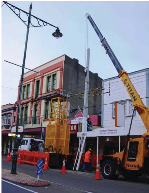
Pole replacement work on a heritage building in Riddiford Street
