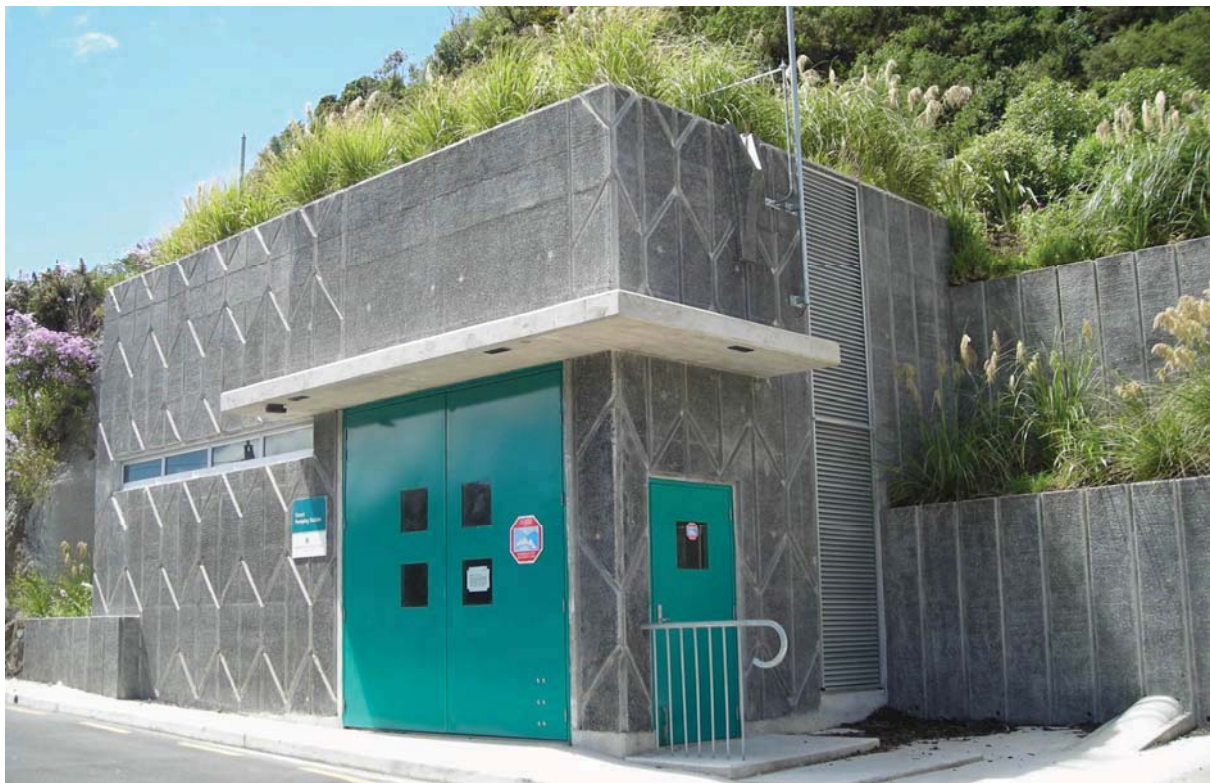
Karori Pumping Station
