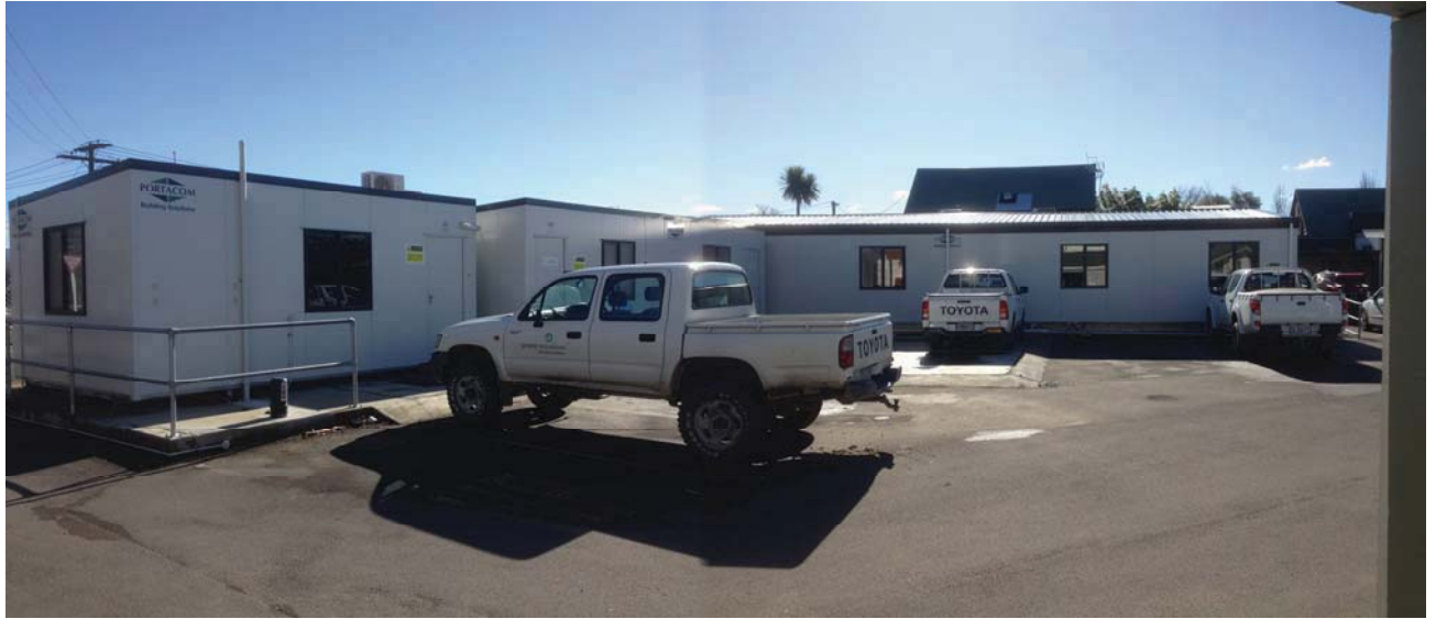
Lab, meeting rooms and office Portacoms at Masterton
