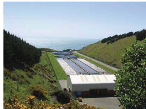
Porirua wastewater treatment plant (photo from PCC website)
