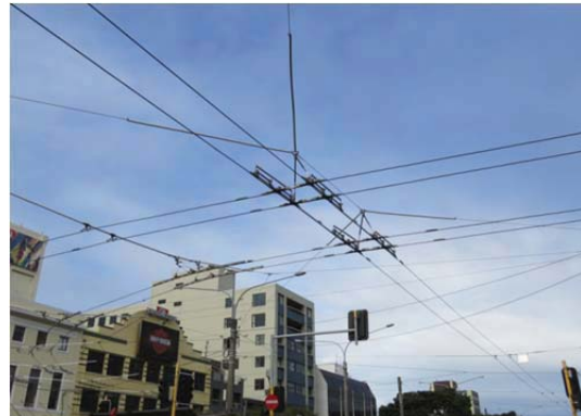
Special works at the junction of Courtenay Place and Cambridge Terrace
