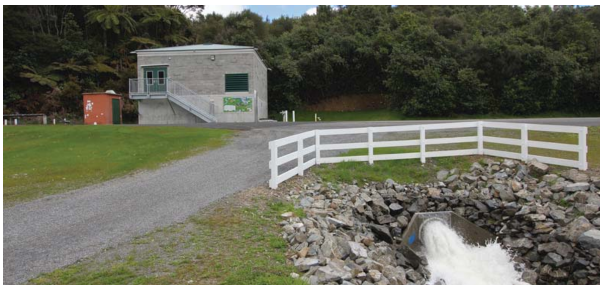
The Wainuiomata hydro-generator building and its Georges Creek outlet
