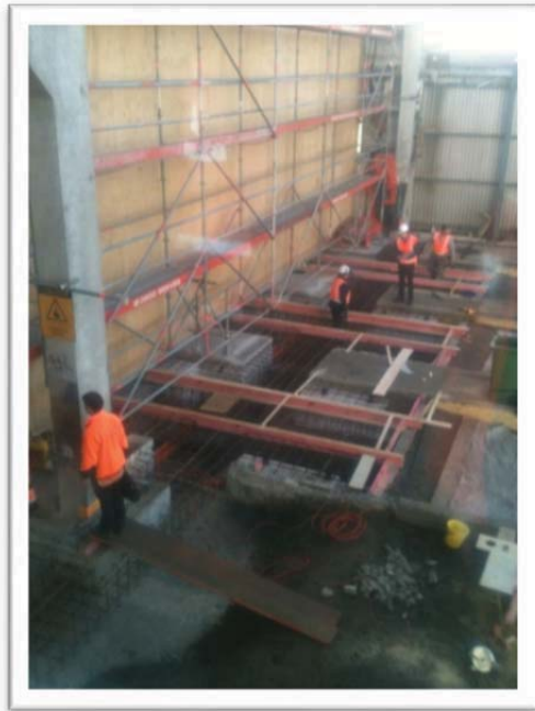
New south wall footing preparation
