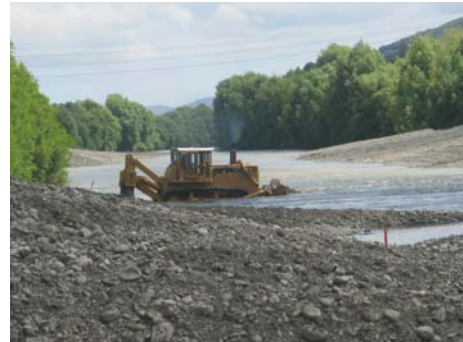
Channel excavation in Hutt River
