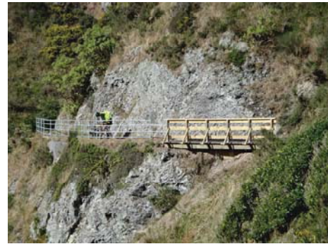
New barrier and bridge on Korokoro Track
