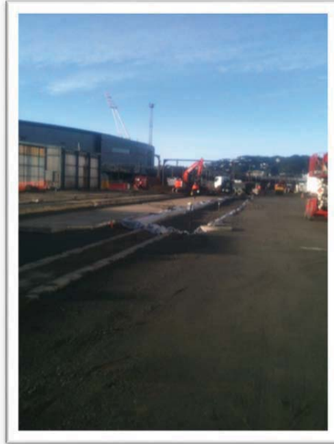
Original 1940's depot area
