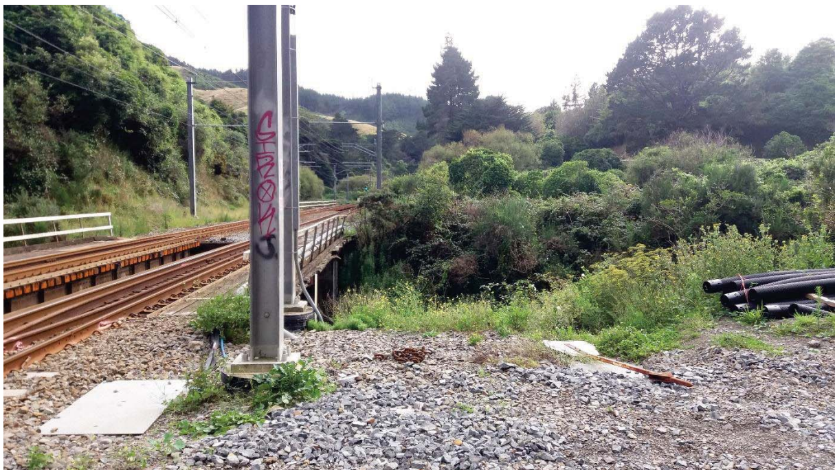
Figure 1: Existing site showing rail bridge adjacent to tunnel portal, looking North
