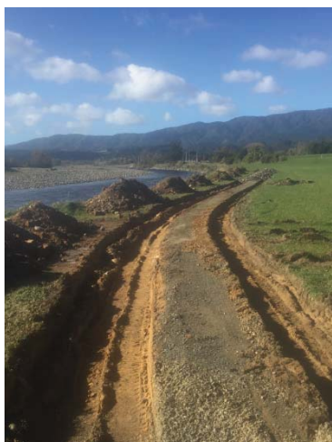
Hutt River Trail widening in progress, Upper Hutt
