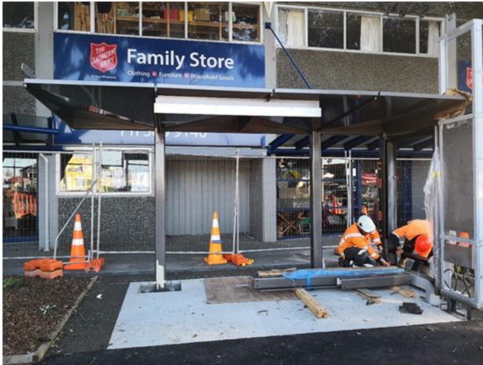
Figure 8 – Shelter Installation – Stop B Mirmar
