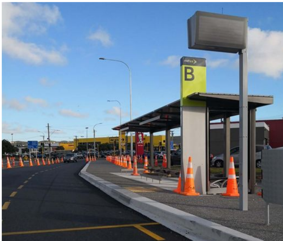
Figure 9 – Large shelter Stop B Kilbirnie
