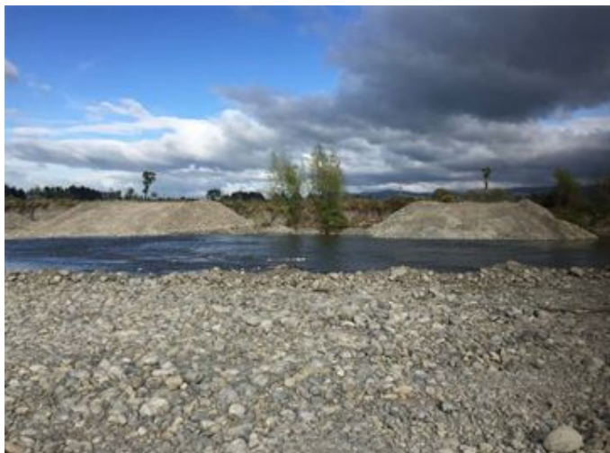
Photo 2: Waingawa gravel groynes and planting
