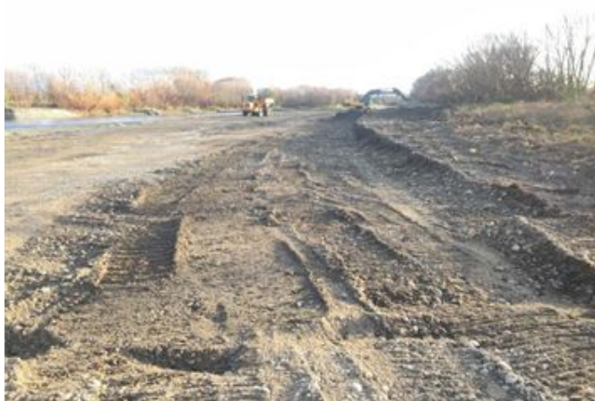
Photo 3: Te Ore Ore gravel extraction from problem beach
