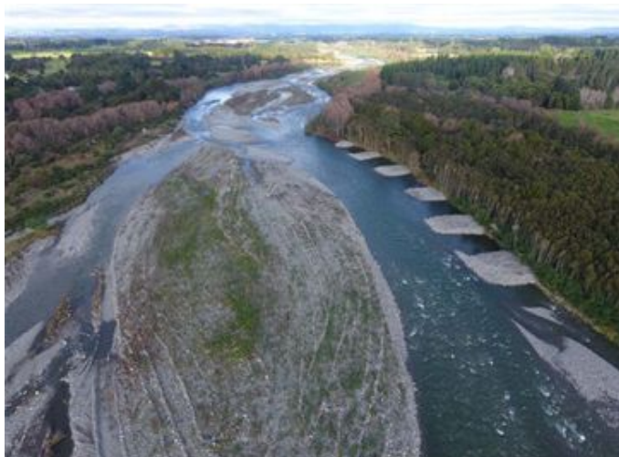
Photo 1: Waingawa gravel groynes at cross section 26
