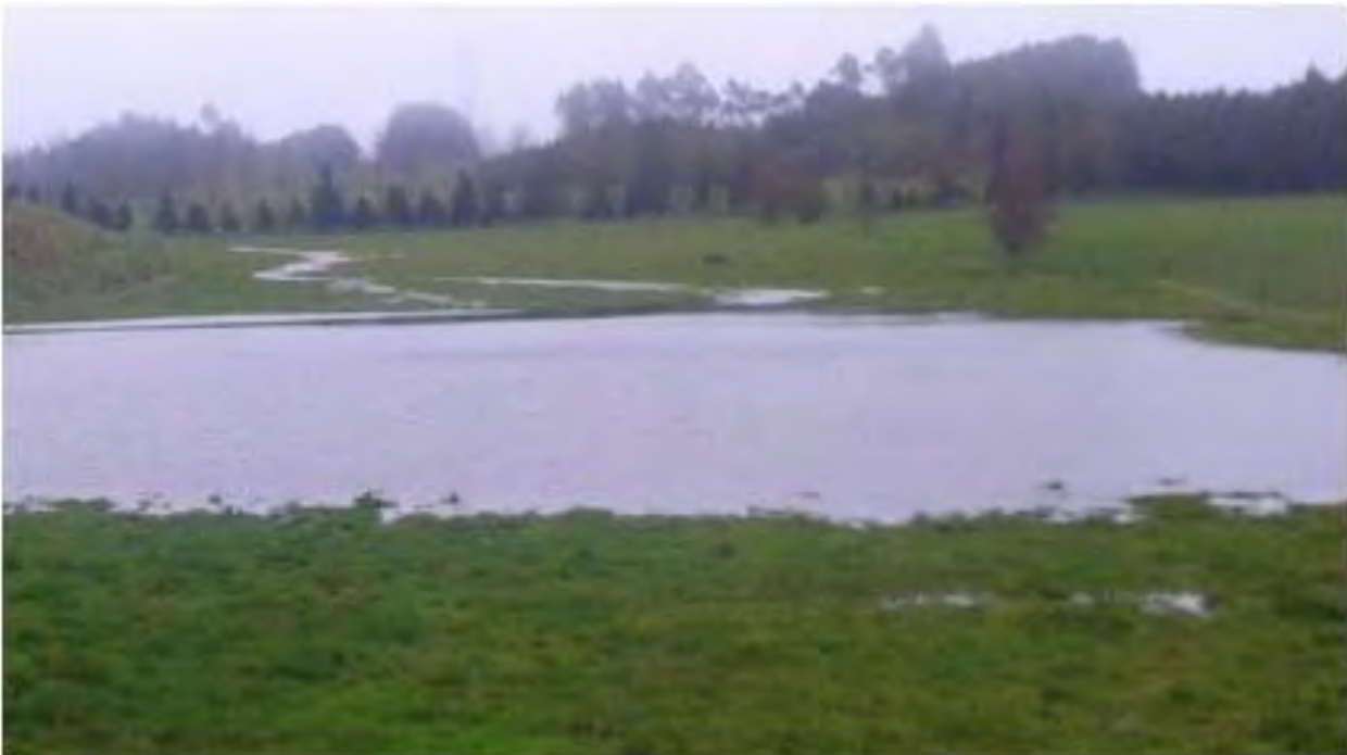
Detainment or detention bunds
