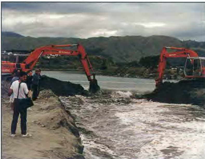
PHOTOGRAPH 8: CUTTING THE WAIKANAЕ RIVER MOUTH, FEBRUARY 1995
