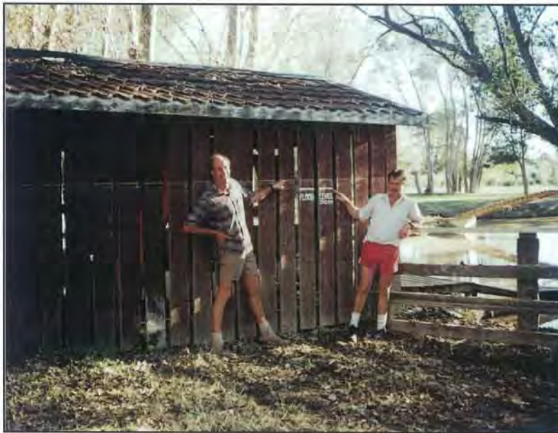
PHOTOGRAPH 3: FLOOD LEVELS FROM THE MARCH 1990 FLOOD ON THE BOATSHED AT EL RANCHO
