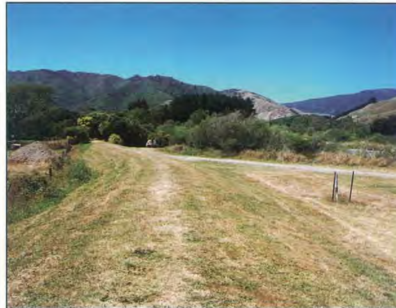
PHOTOGRAPH 4: STOPBANK THROUGH JIM COOKE PARK
