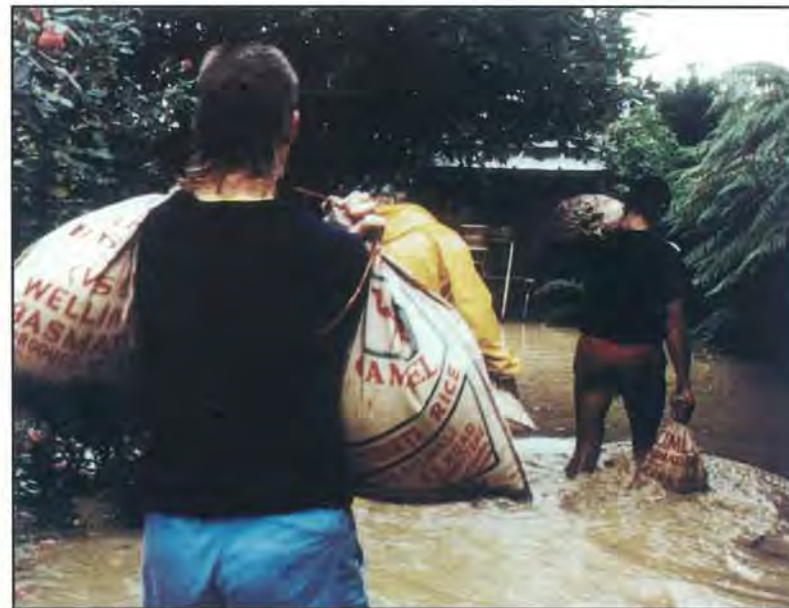
PHOTOGRAPH 6: SANDBAGGING IN OTAIHANGA DURING THE MARCH 1990 FLOOD
