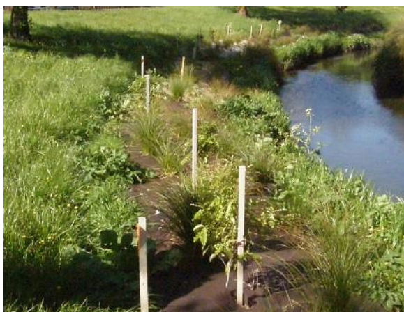
Figure 3 (c). Spray the site with pre-emergent herbicide before planting, to reduce weed competition and maintenance. Use biodegradable weed mat if budget allows (see left). This suppresses weed competition in the first several years while the plants are establishing.
