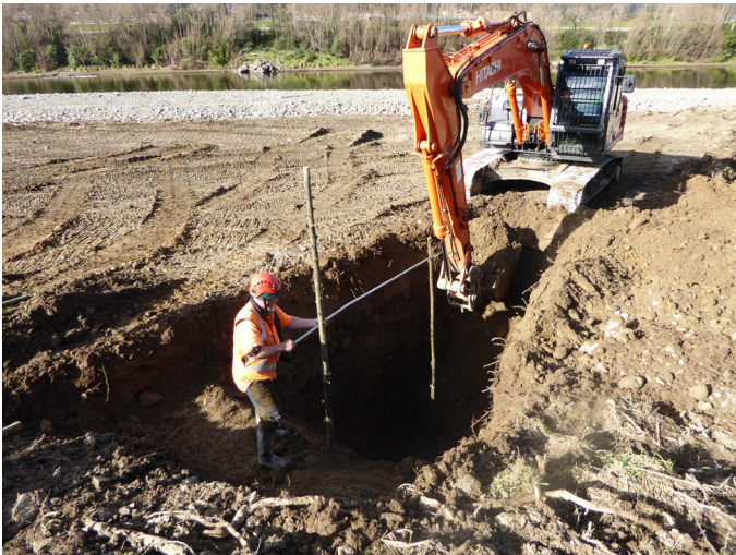
Figure 18: willows will grow from poles driven into the ground with 90-100% success rates, even on sites disrupted by major ground works.
