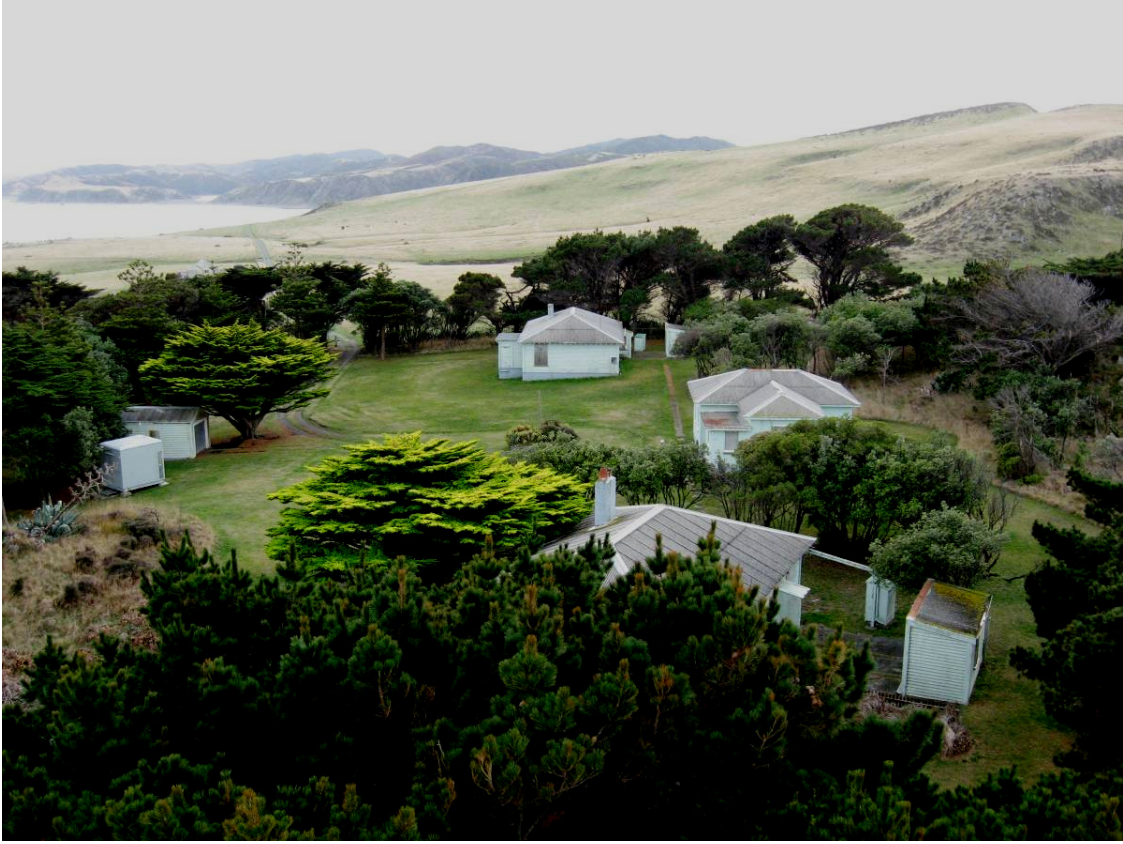
Fig. 8. Keepers' houses and the generator (power) building (centre right) from the south. The garage is at left.
