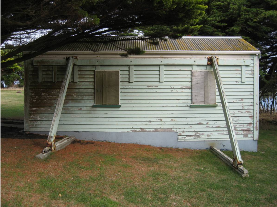
Fig. 14. North elevation of the garage with later buttresses.
