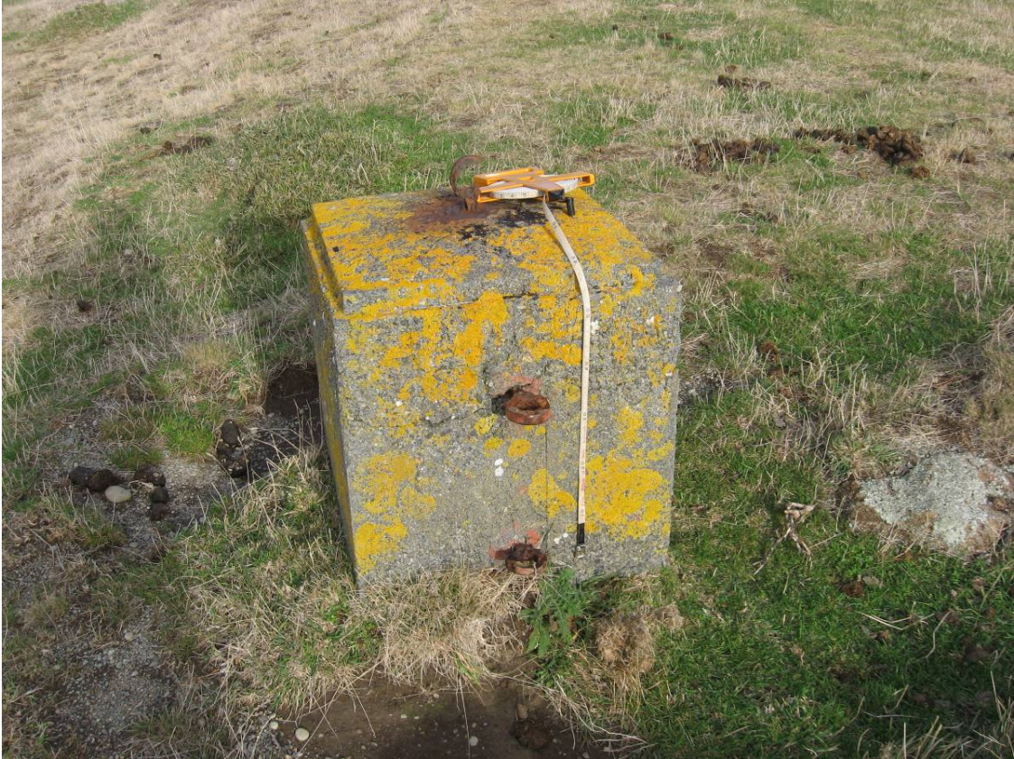
Fig. 18. Concrete counter-weight for the static tensioning stay to the north-eastern mast. It was originally suspended in a steel frame (see Fig. 19).
