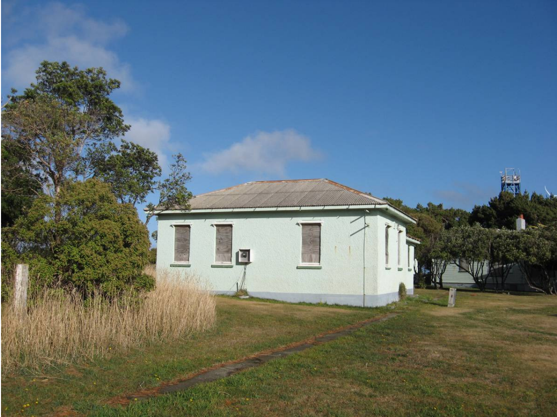
Fig. 13. North elevation of the concrete generator building. Note twin galvanized pipes under the eaves (upper right) which may have held a bracket for the feeder wire to the radio antenna.
