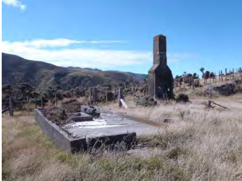
Figure 25: The site of what was the accommodation barracks and ablution block for the men who staffed the observation post. The barracks is assumed to have been constructed of timber and is no longer evident bar the concrete chimney. The ablutions block retains its concrete foundations, floor and drains, but is likewise missing its timber structure.
