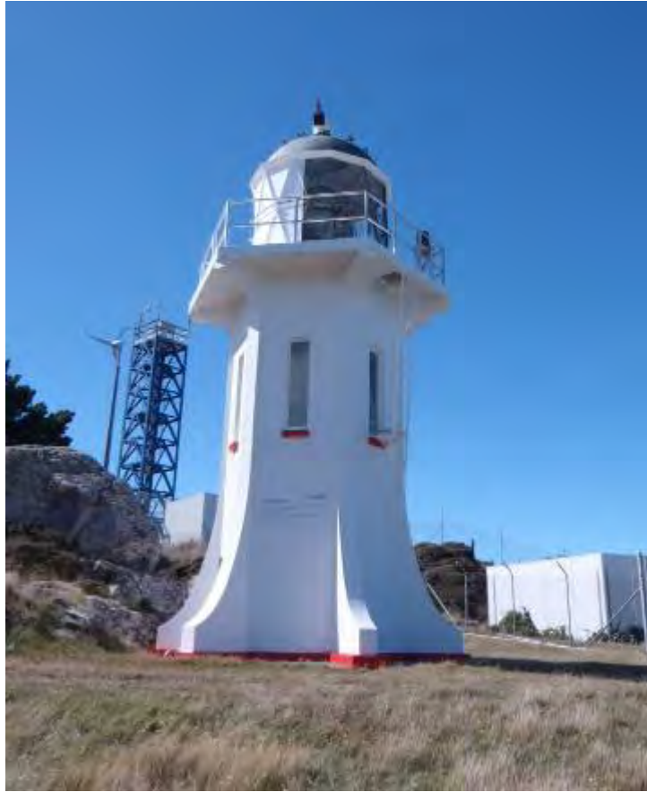
Figure 22: The Lighthouse viewed from the southwest, showing its relationship with the NIWA station behind.
