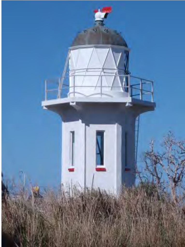
Figure 21: The Lighthouse from the gate at the edge of the accommodation complex.
