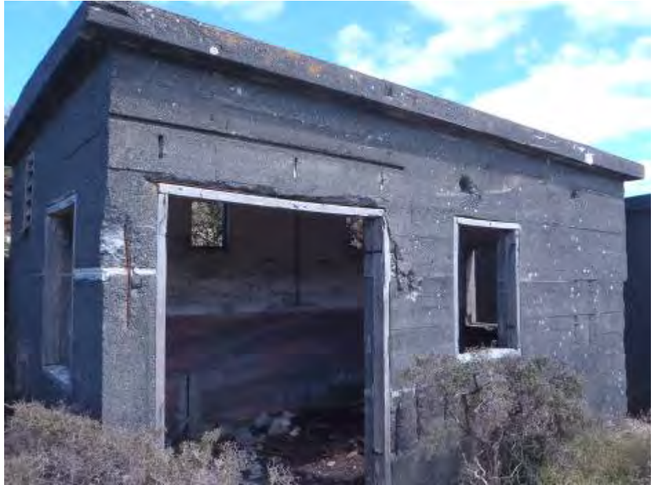
Figure 29: The possible mess room with reinforced concrete walls.
