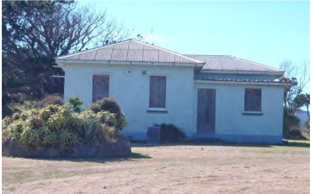
Figure 17: Diesel generator building with circular garden in the foreground.
