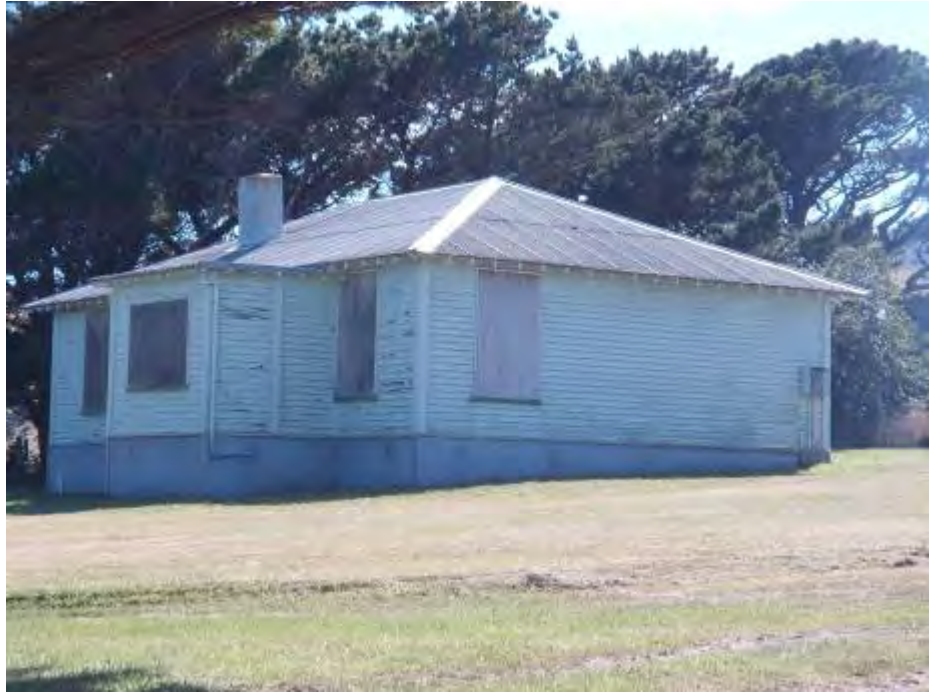
Figure 19: Number Two Lighthouse Keepers' House showing the additional bedroom on the front elevation of the house.
