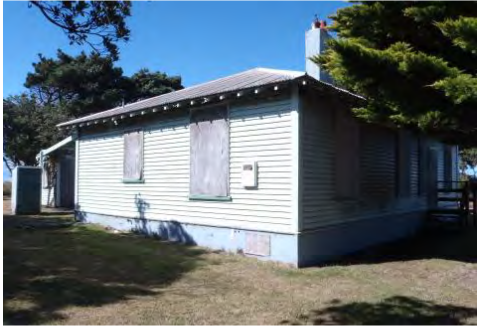
Figure 15: Number One Lighthouse Keepers' House from the southeast, with outhouse and pump house visible at the rear.
