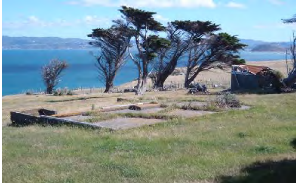
Figure 23: Foundations of the WAAC barracks.
