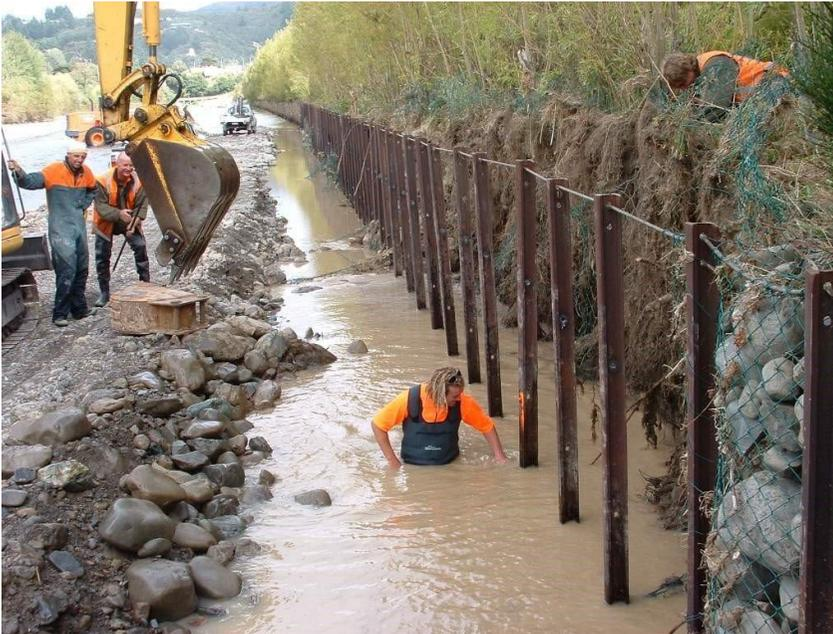
*Formation of gabion structure; note separation of works from flowing channel and machine operating out of the water*
