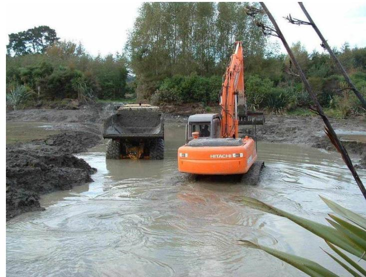
*Silt excavation in Chystalls Lagoon. Note use of self-draining weed bucket*
