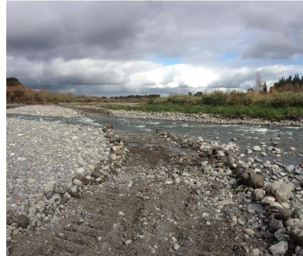
*Temporary vehicle access track on river bed, formed by blading with a bulldozer*
