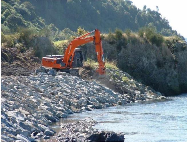
*Maintenance – repairs to rock lining. Note platform formed in riverbed as machine is unable to work from the bank edge to rebuild this section of lining*
