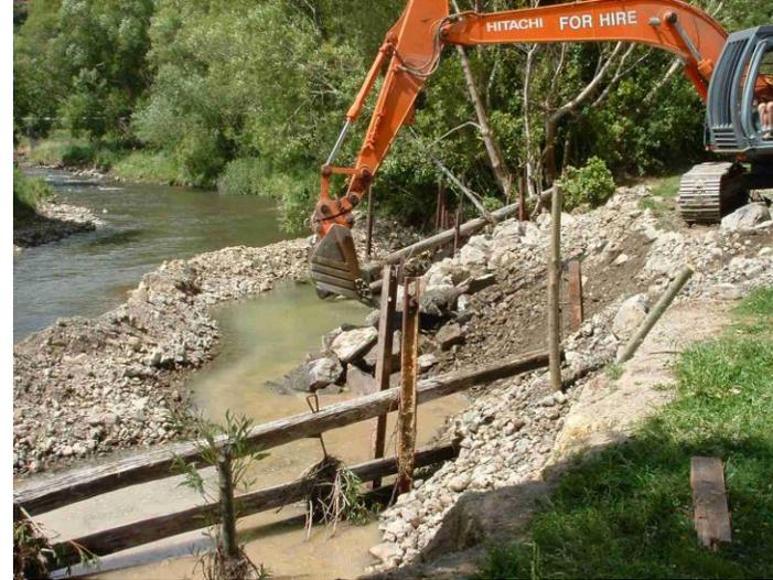
*Repairs to timber permeable groynes on the Wainuiomata River. Note the separation of the work area from the wet channel through the use of bunding*
