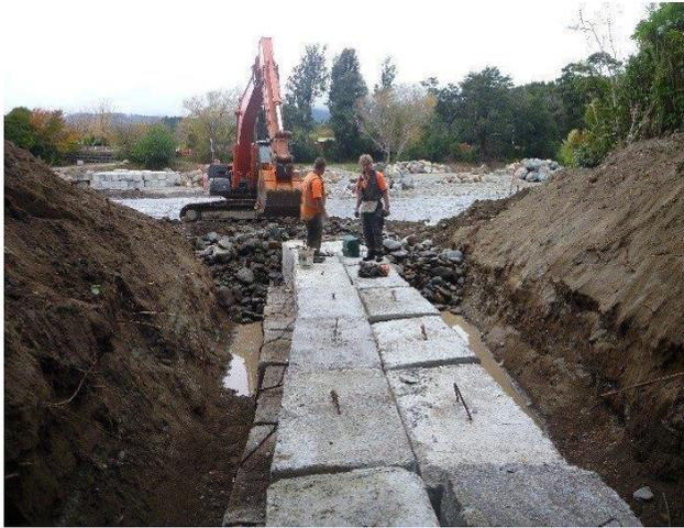
*Foundation excavated and groyne core of concrete blocks placed out of flowing water*
