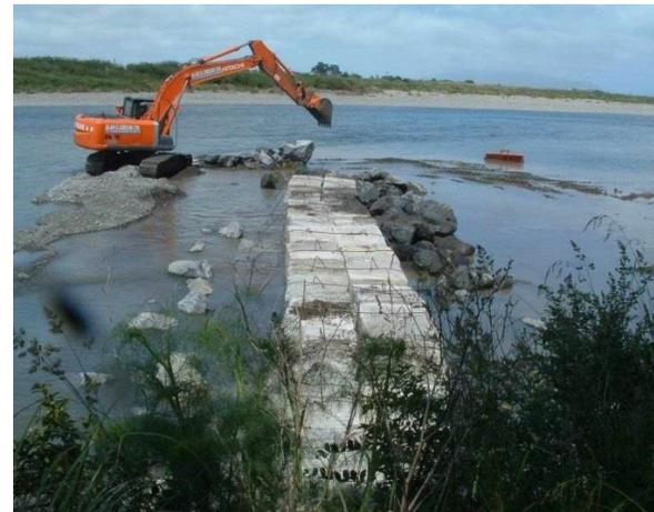
*Groyne construction, showing use of bunding to protect works from flowing water and use of a formed working platform to elevate machinery out of flowing water*
