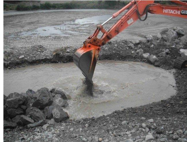
*Excavating trench for foundation rock with machine located out of flowing water*
