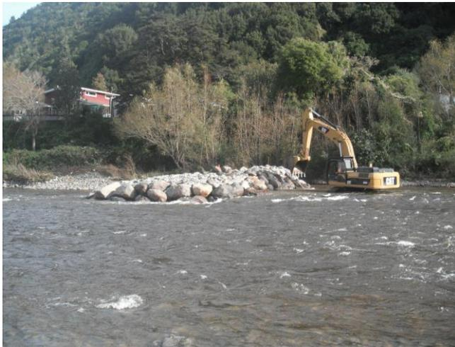
*Groyne placement. Machinery working close to bank edge to minimise disturbance to the riverbed*
