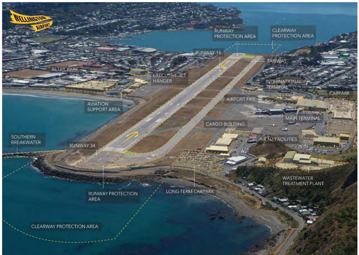
Figure 2: Current configuration of Wellington International Airport, Source: Assessment of Environmental Effects , Mitchell Partnerships, 28 April 2016, P.27
