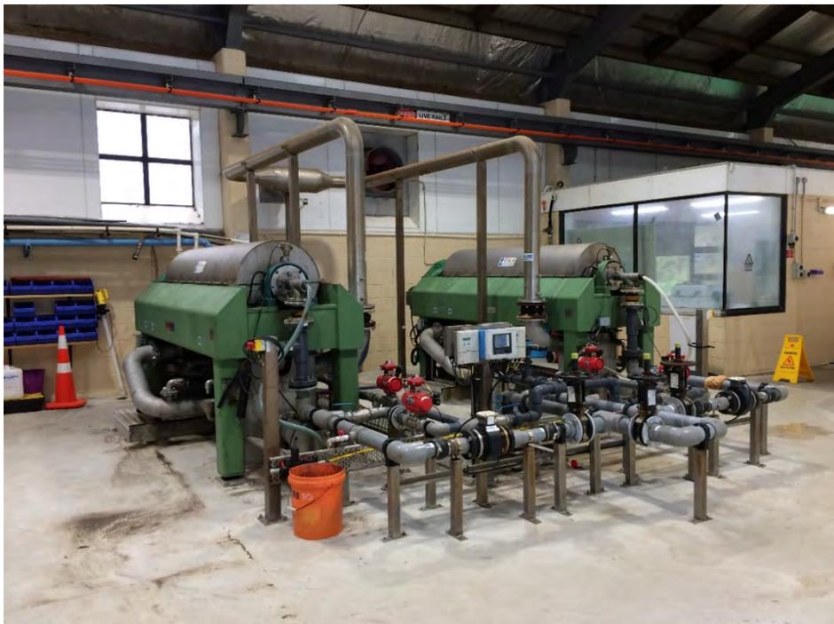
**Figure 8: Sludge dewatering centrifuges**
