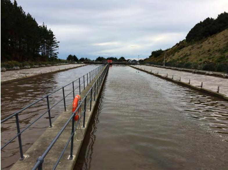
**Figure 10: Aeration basin, with turbulence from active aeration being apparent in the side channels**
