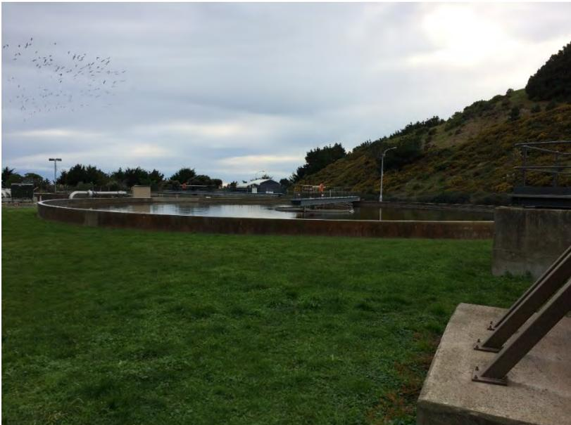
**Figure 11: One of the three clarifiers used to settle remaining solids from the wastewater effluent prior to UV treatment and subsequent discharge via the ocean outfall**
