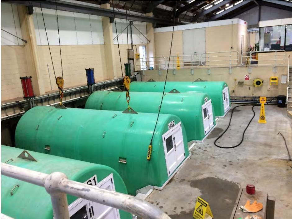
**Figure 7: The Milliscreening Hall, with fibreglass covers over the screens to minimise H<sub>2</sub>S/ odour release**
