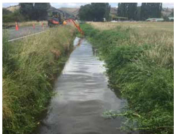
Good practice: The vegetation on both banks has been left untouched by the excavator.
