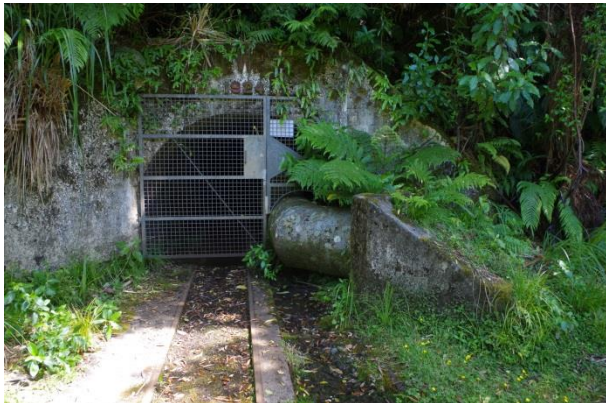
Main tunnel, south-eastern portal with in situ tram rails
