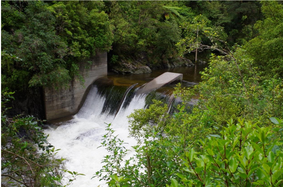
Weir and intake (S26/4) viewed from track to southeast, the true right abutment contains the entrance to the pipeline tunnel
