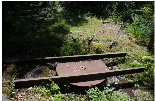
Tram way turntable in front of SE portal of main tunnel
