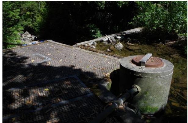
Big Huia intake looking across the top of the intake structure
