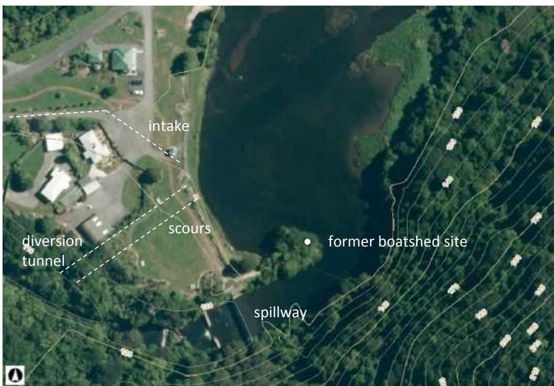
Aerial photography with contours showing the Wainuiomata waterworks dam with spillway to the south, and former location of the boatshed on the narrow headland jutting out into the reservoir. Intake, scours and diversion tunnels indicated with dotted lines (Source Hutt City Council, on-line GIS, 2015)
