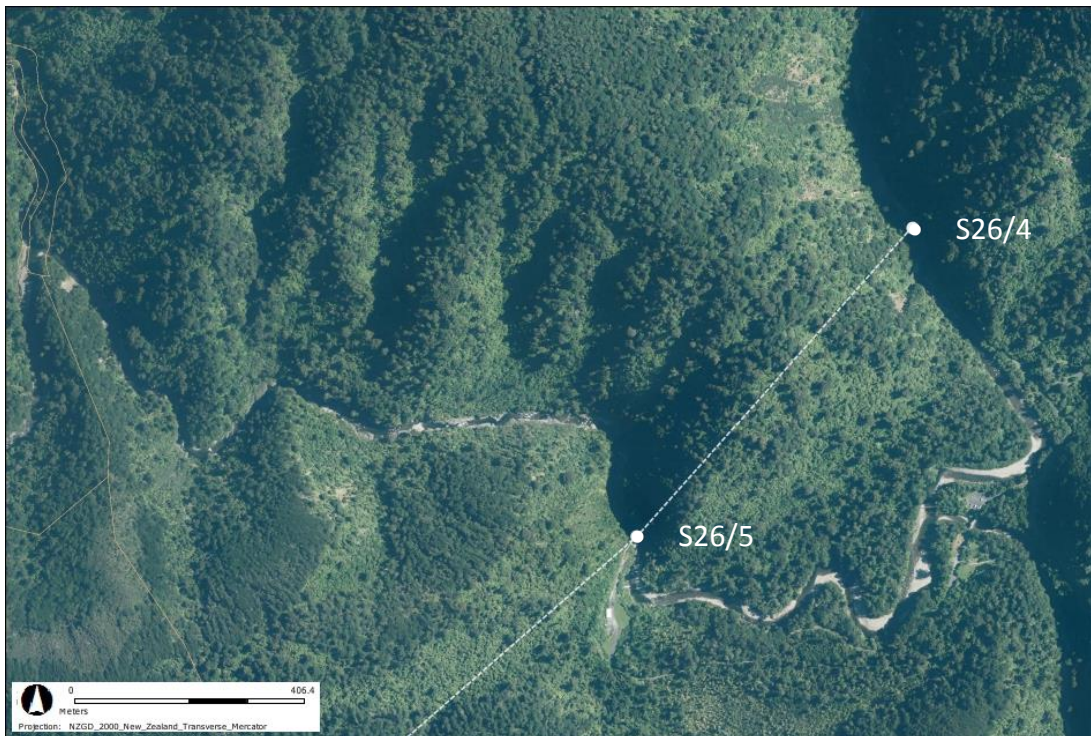
Aerial photography showing the location of the intake (S26/4) and pipe bridge (S26/5) associated with the Kaitoke water supply. Direction of pipeline shown as dotted line (Source Upper Hutt City Council on-line GIS, 2015)
