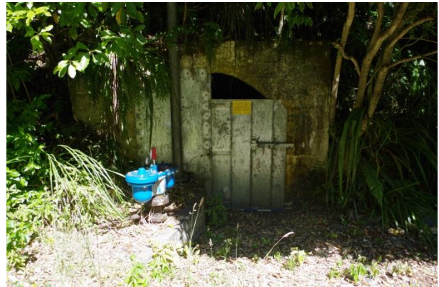
Short tunnel, western portal
