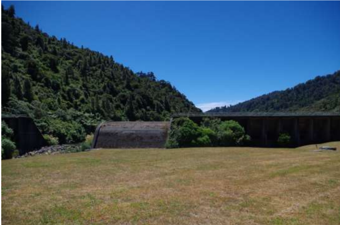
Morton Dam viewed from western downstream side. Demolished section and spillway visible in the left of frame (Dodd, 2015)
