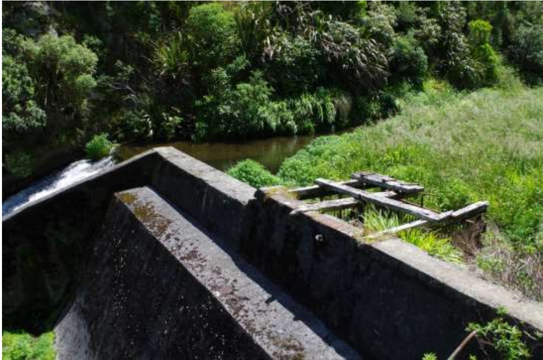
Looking southwest over the Petone Woollen Mill's weir. Intake in foreground to right of frame, spillway in background to left (Dodd, 2015)
