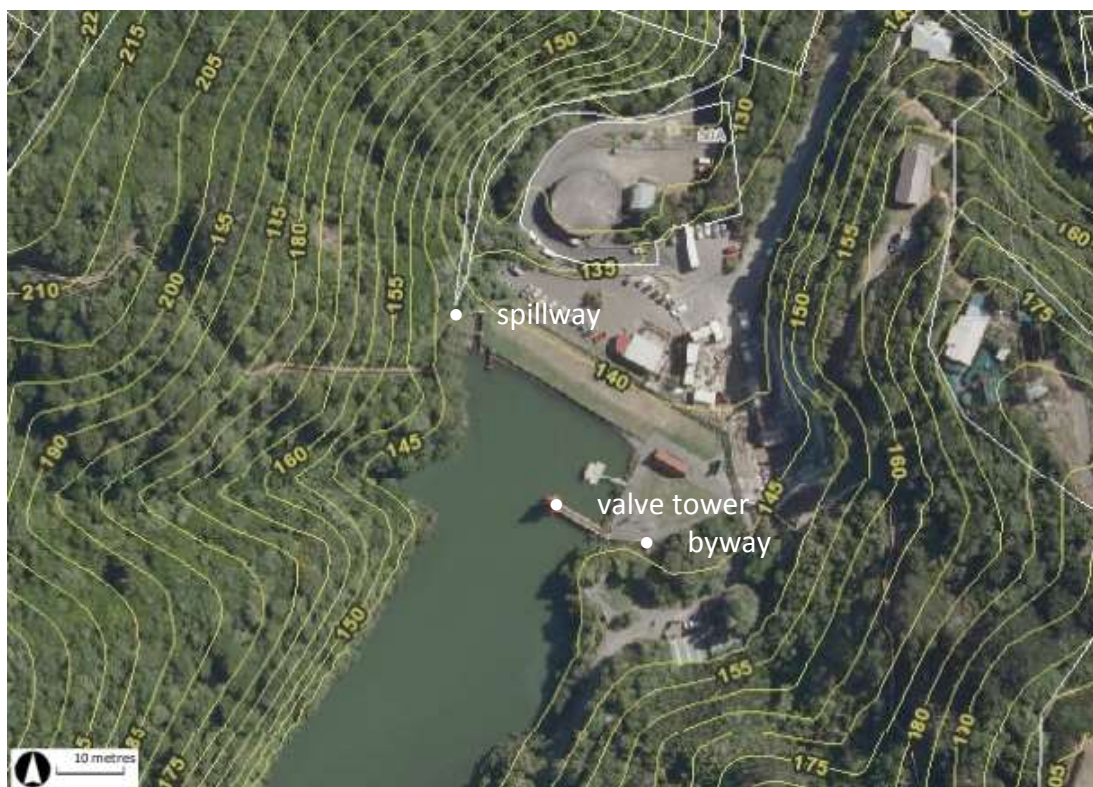
Aerial photography with 5-metre contours showing location of dam, western spillway, valve tower and start of eastern byway (Source Wellington City Council, on-line GIS, 2015)
