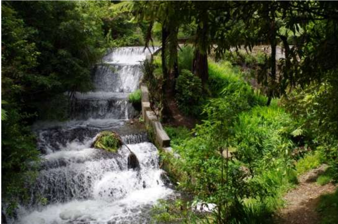
Looking east from the bottom of the Korokoro dam spillway (Dodd, 2015).
