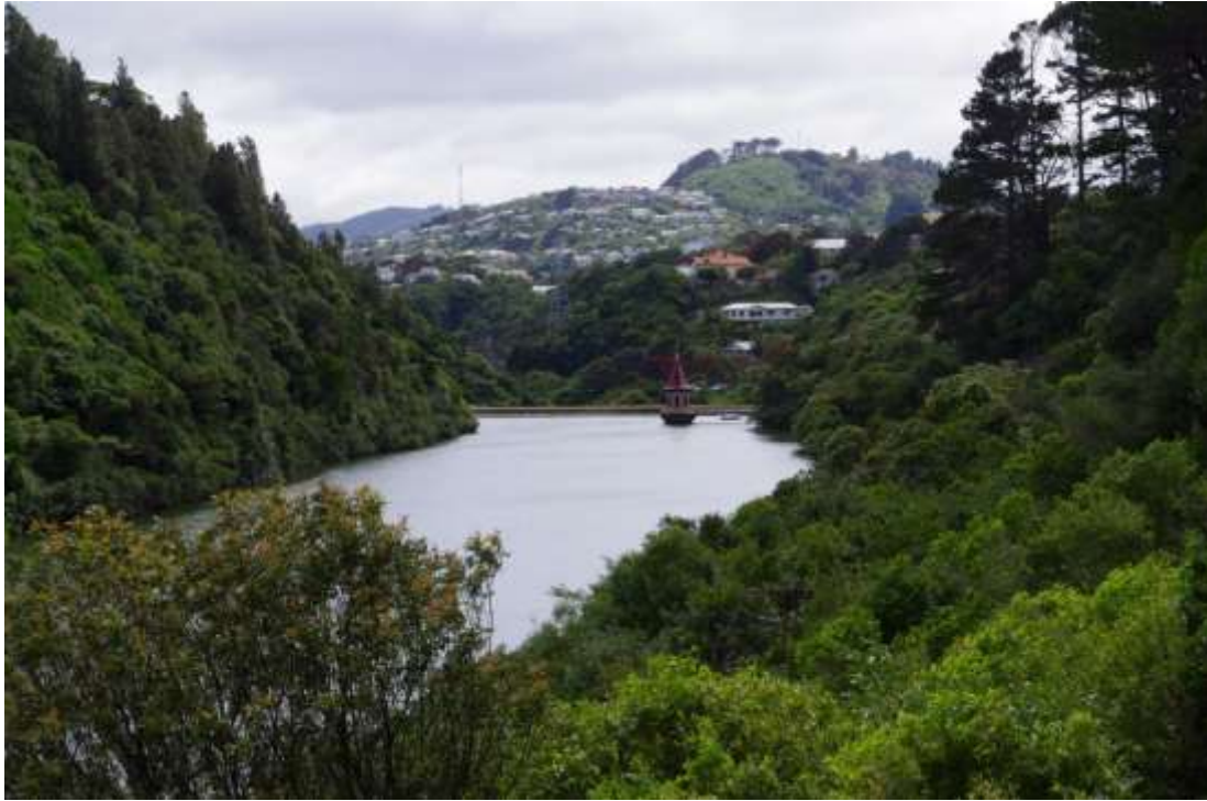
Lower Karori Dam and reservoir viewed from the south (Dodd, 2015)
