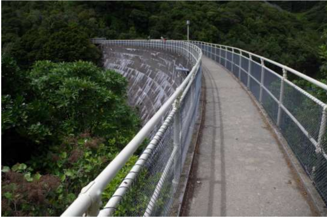
Looking east along the top of the Upper Karori dam (Dodd, 2015)
