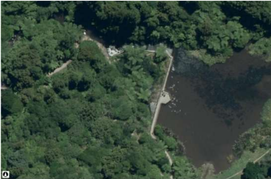
Aerial photography showing Korokoro dam and spillway (Source Hutt City Council on-line GIS, 2015)
