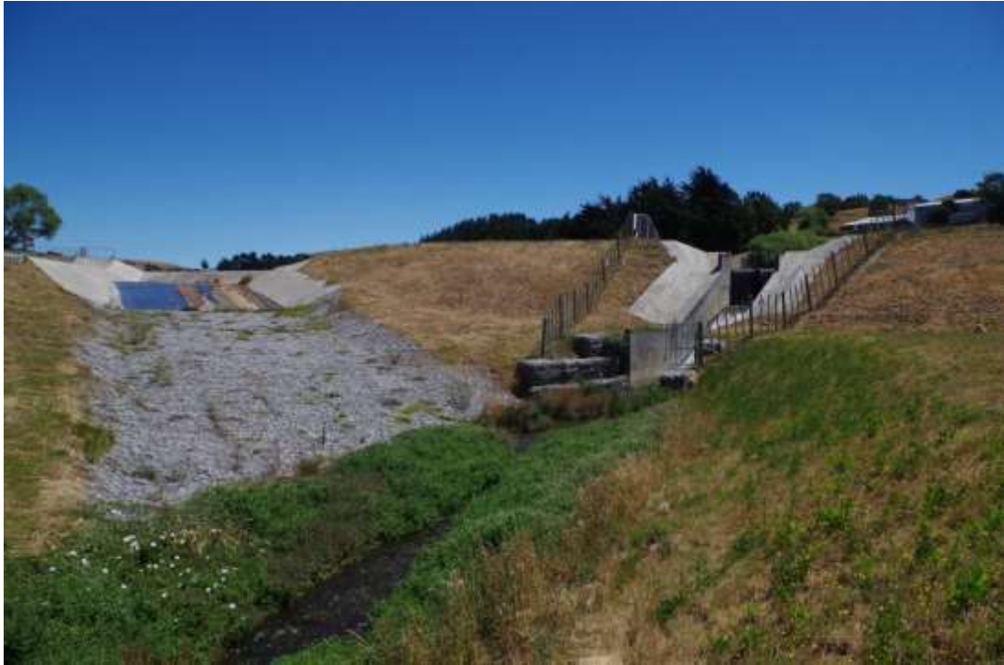
Upper reservoir dam and spillways (Dodd, 2015)
