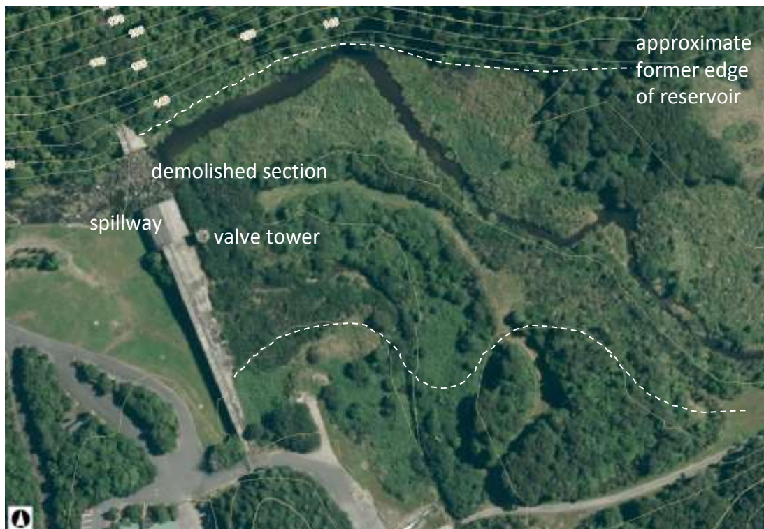
Aerial photography with contours showing location of Morton dam, approximate former edge of the reservoir, spillway, valve tower and demolished section of dam in stream bed (Source Hutt City Council, on-line GIS, 2015)
