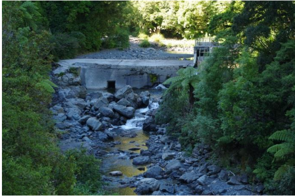
Main weir viewed from downstream side to NNW
