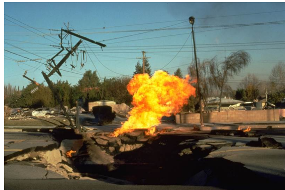
Above: A gas main ruptures in the 1994 Northridge earthquake.
