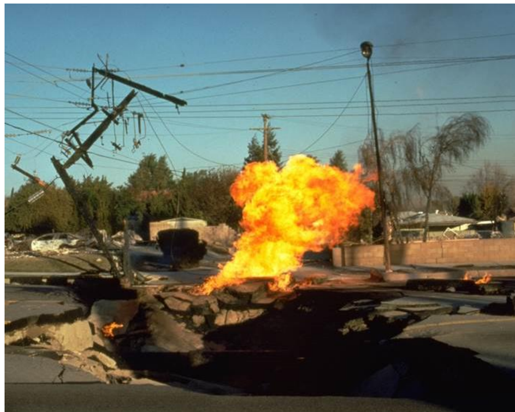
Above: A gas main ruptures in the 1994 Northridge earthquake, USA.
