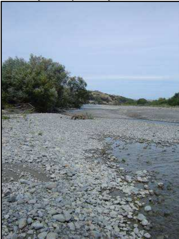
Channel realignment work attempts to maintain central alignment
