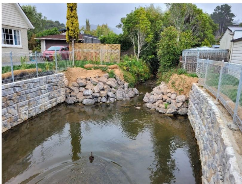
*Figure 7 Redi-Rock walls and scour protection upstream of Sunbrae Culvert (photo credit: GHD)*
