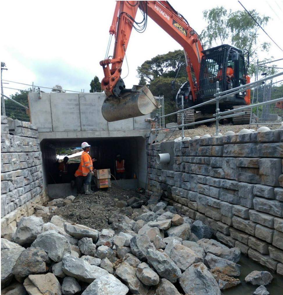
Figure 8 Placement of stream bed material within Pinehaven Culvert using conveyors (photo credit: GHD)
