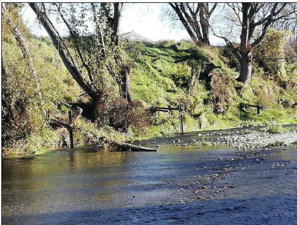
Figure 7-12 – Railway groynes and vegetation on the true right bank in the vicinity of the debris recording location
