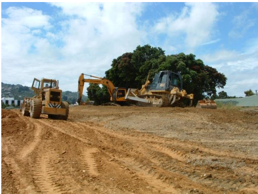
Strand Park Stopbank Construction February 2009
