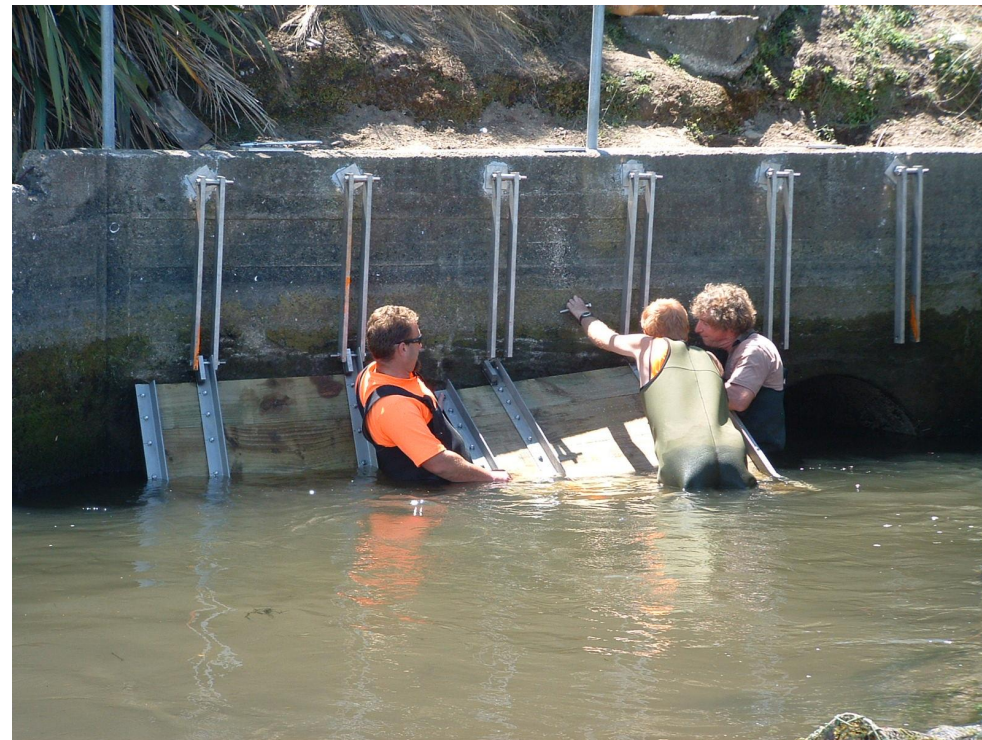
Installing Te Mome floodgates
