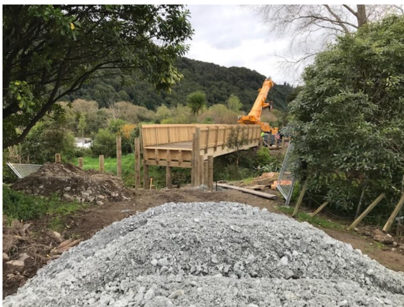
Figure 5: Hulls Creek Bridge under construction
