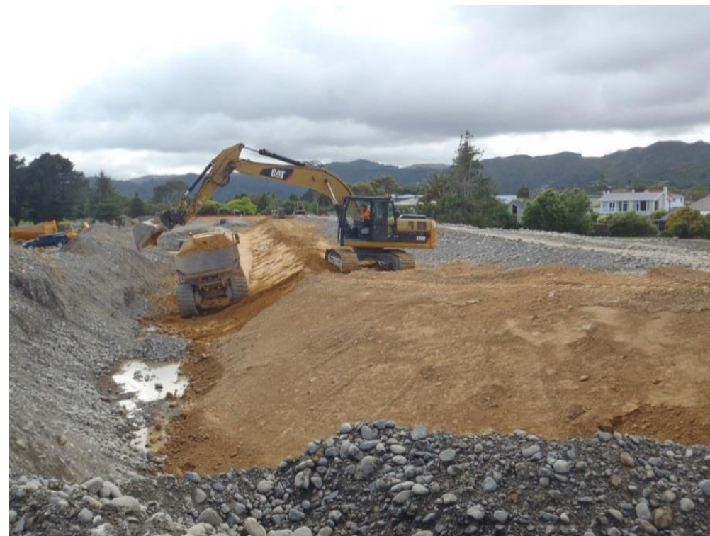
Boulcott Stopbank Construction November 2012
