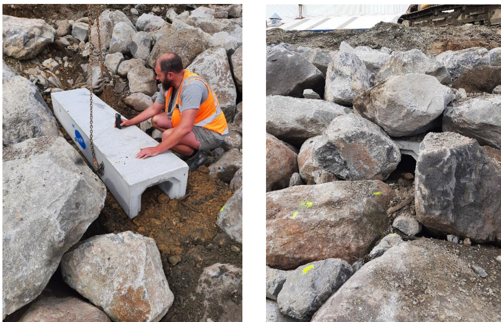
Figure 1: Construction of penguin motels at Site 11
