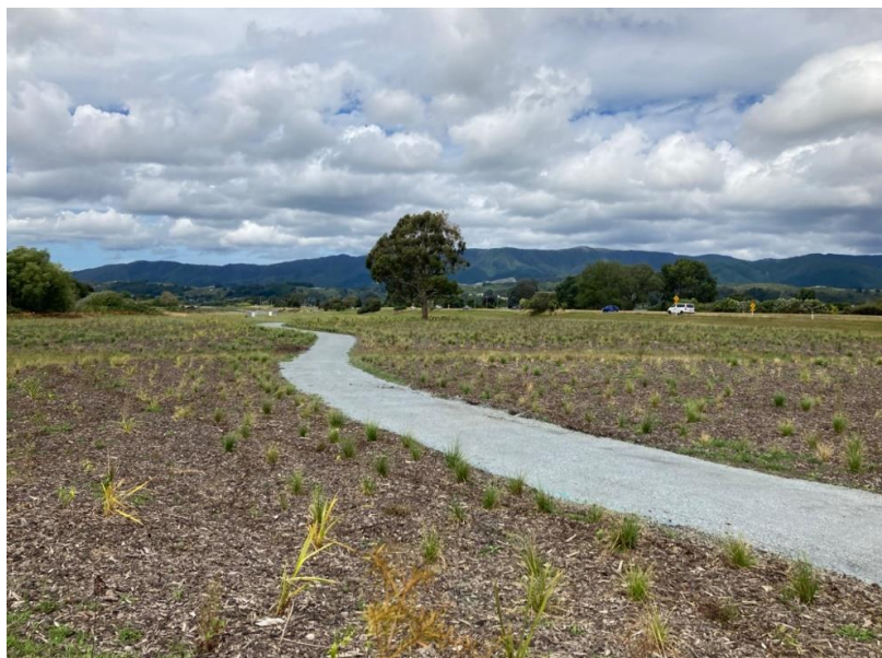
Figure 4: Poets Park planted area and track under construction
