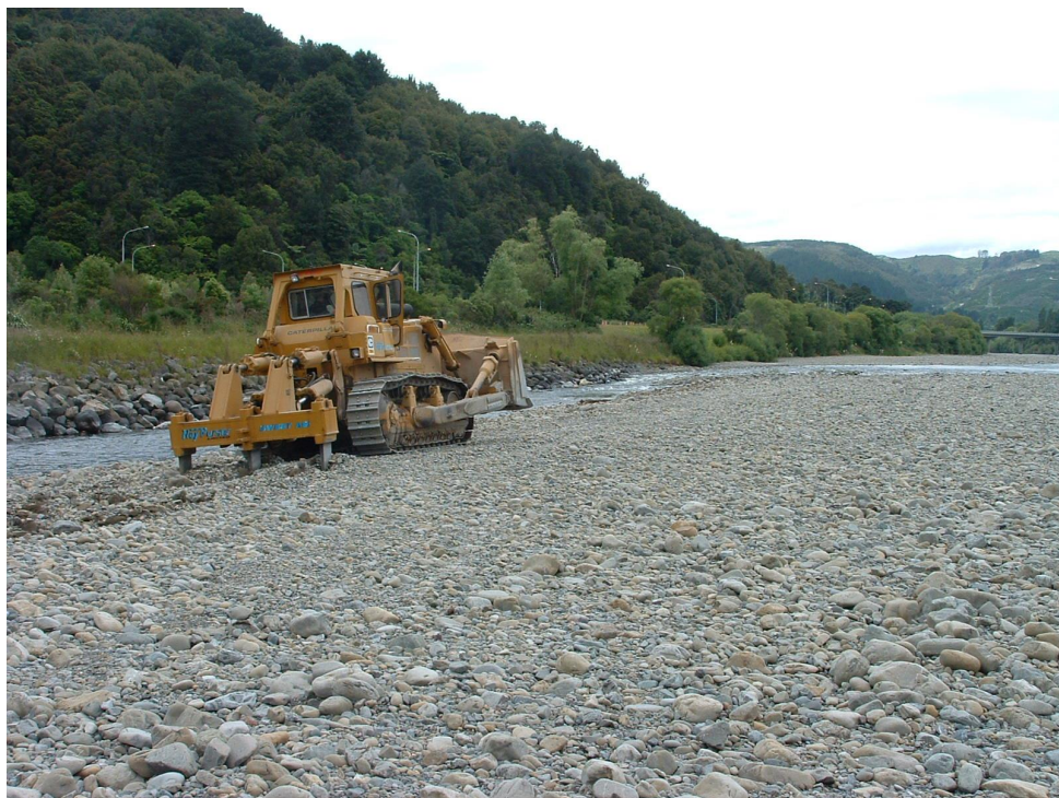
Beach ripping, Trentham Memorial Park
