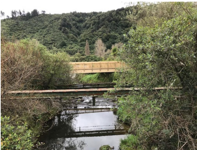
Figure 6: Hulls Creek Bridge in place
