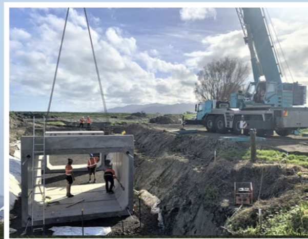
Above: Culvert crossing construction
