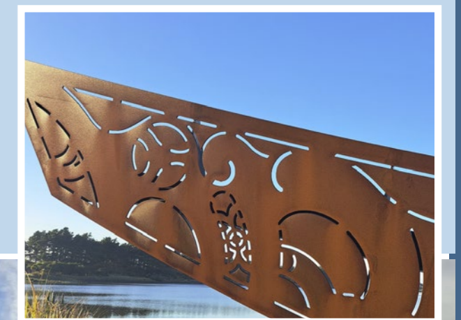
Mahi Toi designs associated with the pump station are integral to the wider Stead Street climate resilience project. The above image shows the design detailing at the end of the new sheet pile wall, conceptually transforming it into a Waka Tiwai.
