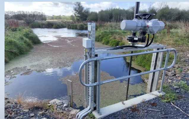
The flow gate and its solar powered actuator valve. Photo: ORC/Tim Ware
