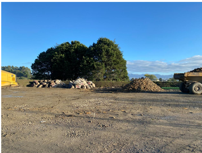
Figure 9: Stage two – Secondary stockpile site adjacent to the Riverside Cemetery
