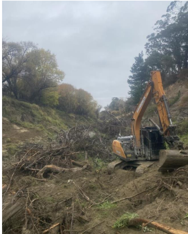
Figure 4: Whareama River – blockage removal commenced
