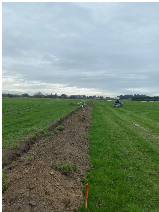
Figure 16: Daleton Nursery irrigation construction underway
