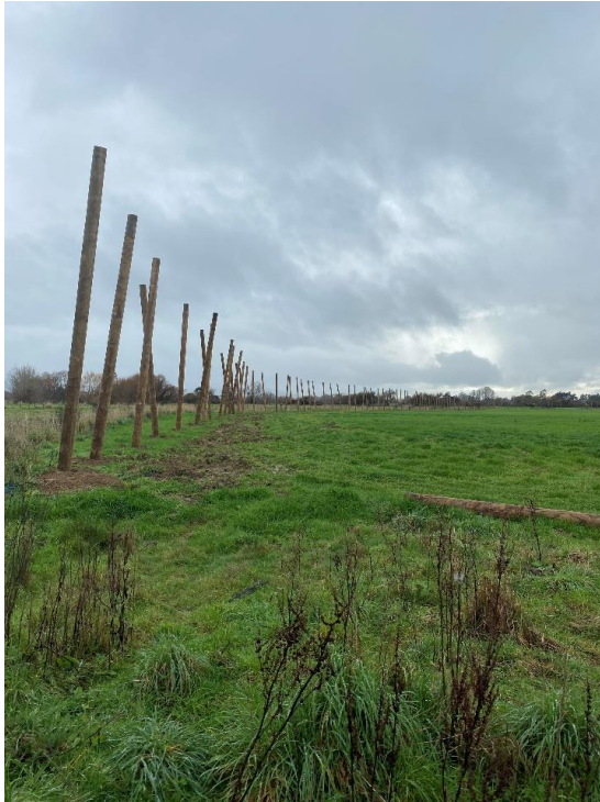
Figure 15: Daleton Nursery 6m artificial shelter construction
