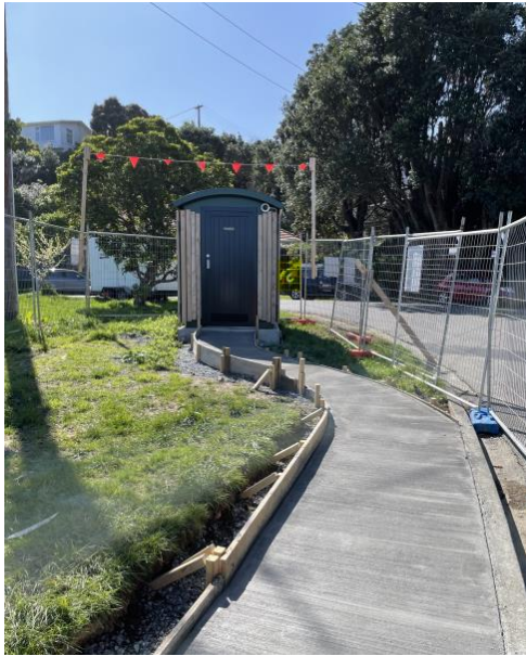
Image 1: Facility – installation in progress (Darlington Rd)
