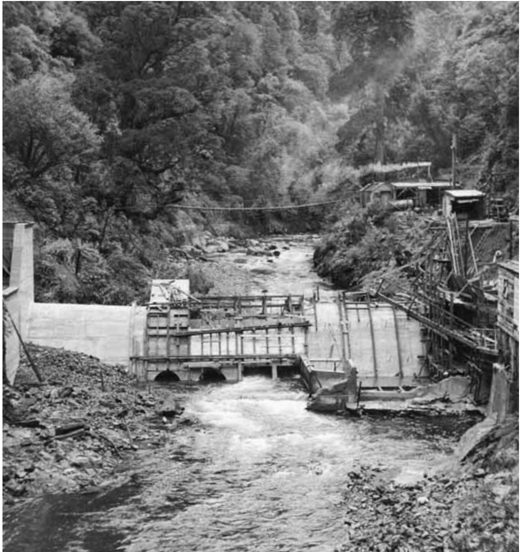
Kaitoke Weir construction
