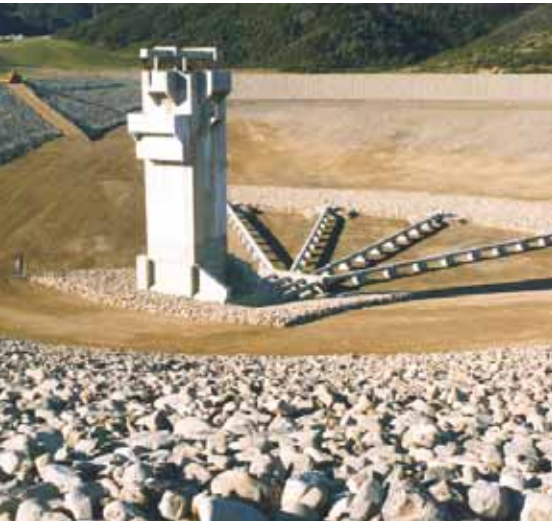
Building the Te Marua storage lakes, 1987
