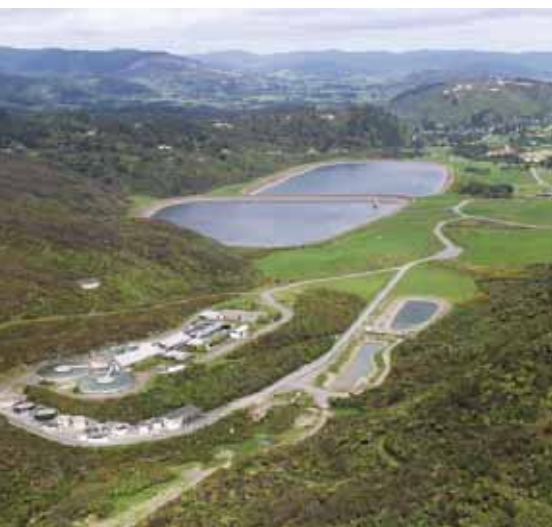
Aerial view of Te Marua storage lakes and water treatment plant
