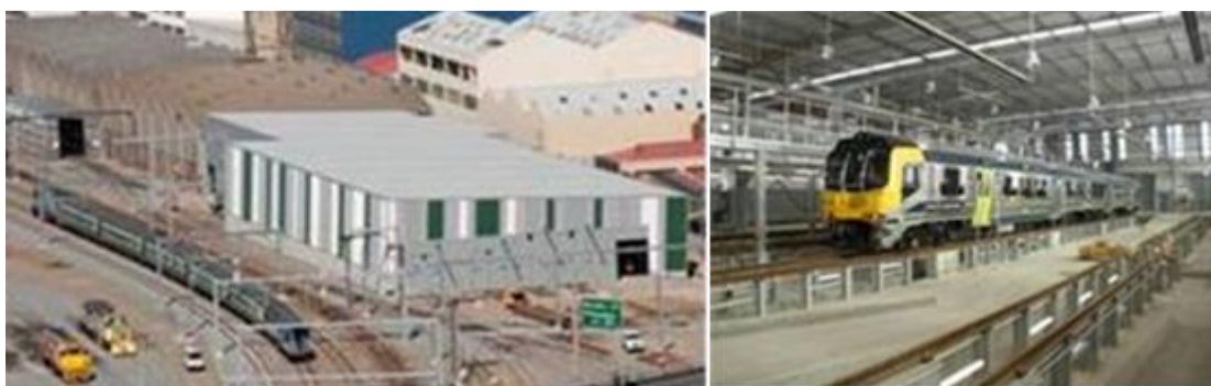
Figure 67: EMU maintenance depot facility
