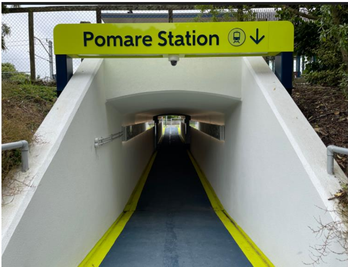
Figure 40: Upgraded Pomare Station subway
