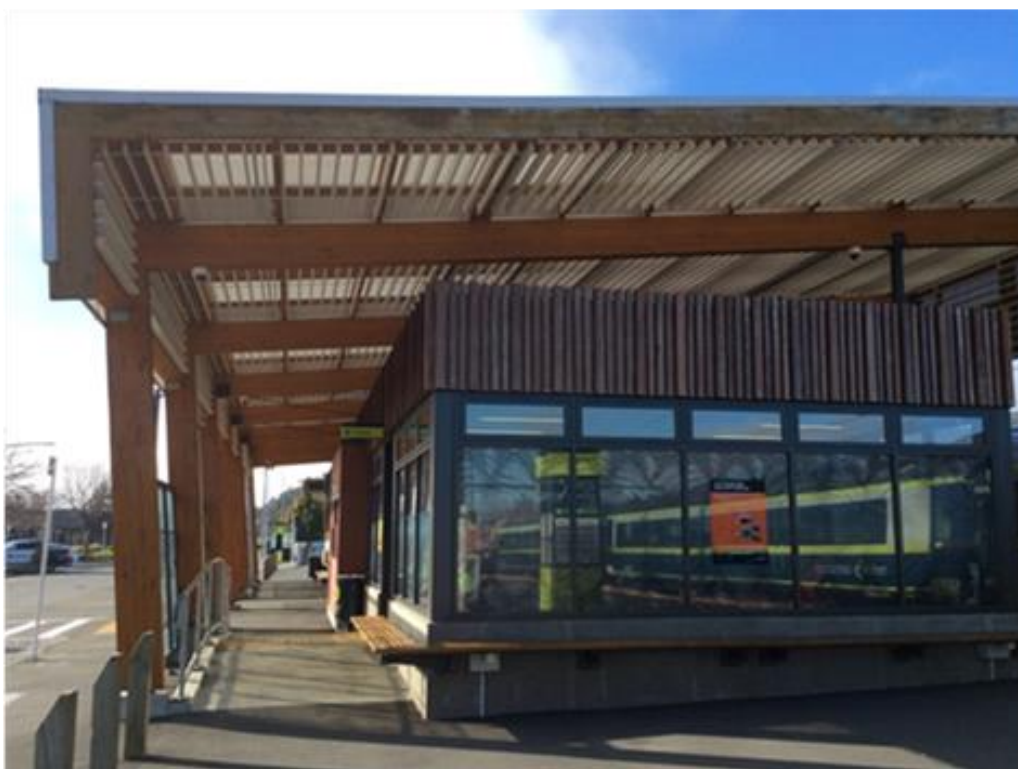
Figure 33: Upper Hutt Station Building – rebuilt in 2015.
