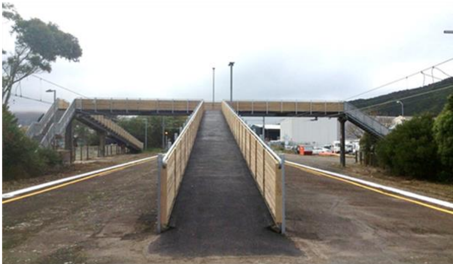
Figure 62: Wingate North pedestrian overbridge – post seismic strengthening improvements
