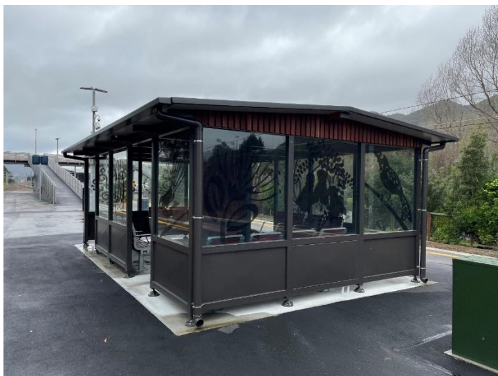
Figure 36: New Wingate shelter
