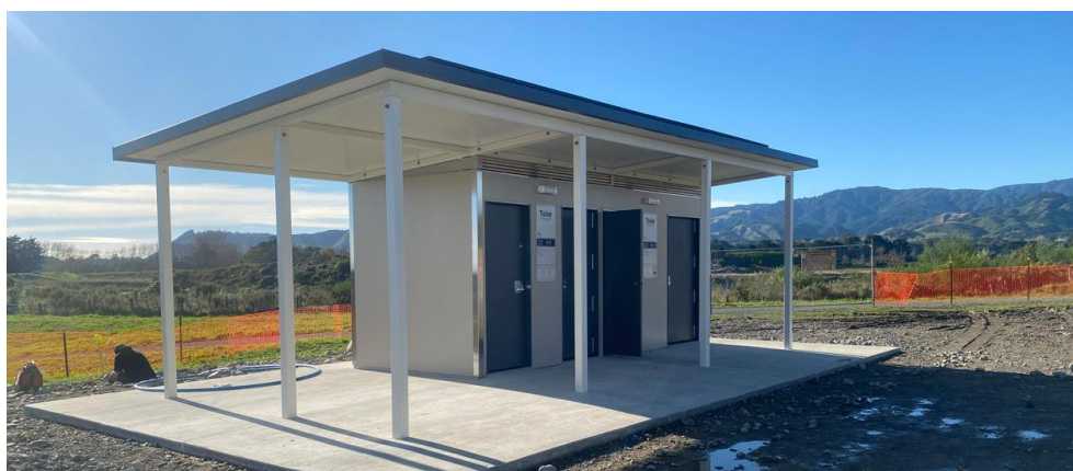
Image 8: Toilet prefab building in place - pre landscaping (13.06.2024)
