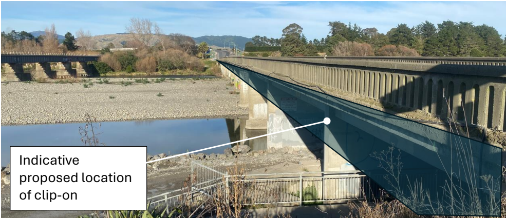
Image 6: Old SH1 bridge – before clip on path is added
