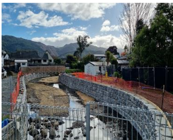
Image 1 Looking downstream from Sunbrae Dr. towards pedestrian bridge (photo credit: GHD)
