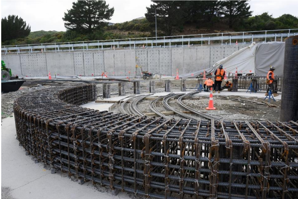
Figure 11: Porirua Wastewater Retention Tank Construction
