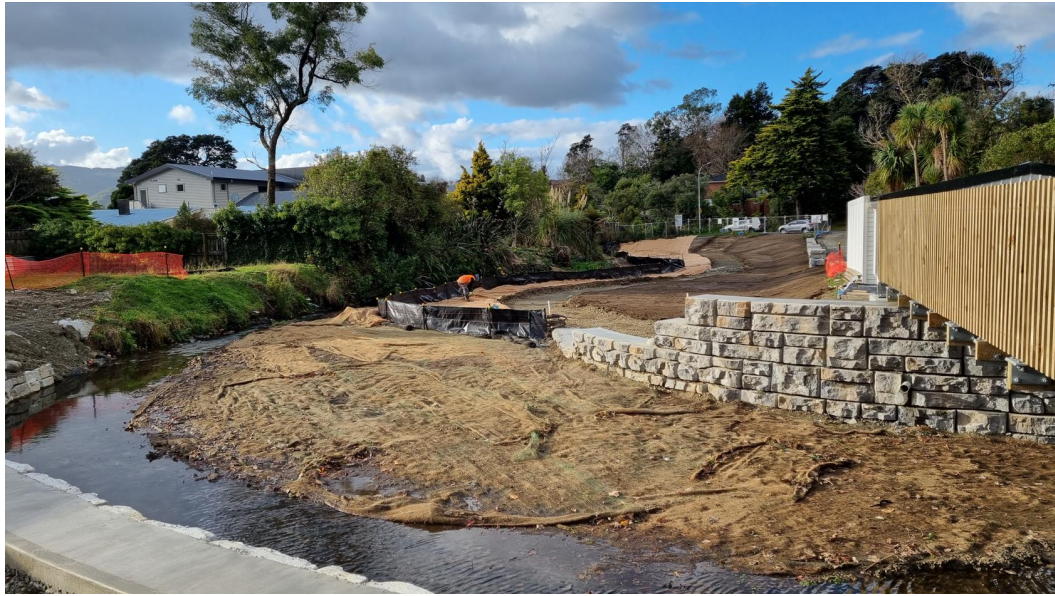
Image 3 Pinehaven Stream siteworks looking downstream from pedestrian bridge (photo credit: GHD)
