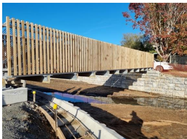
Image 2 Pedestrian bridge installed on concrete foundations (photo credit: GHD)
