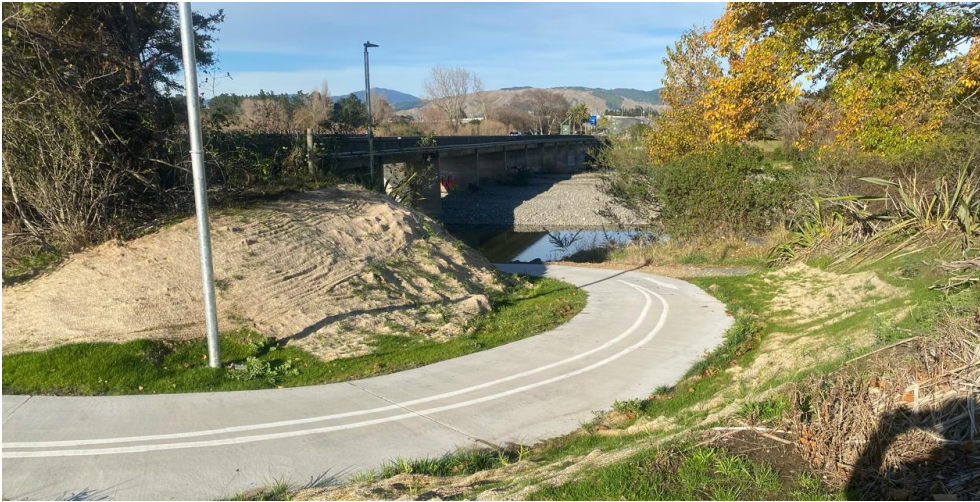
Image 5: New NZTA track around and under old SH1 bridge
