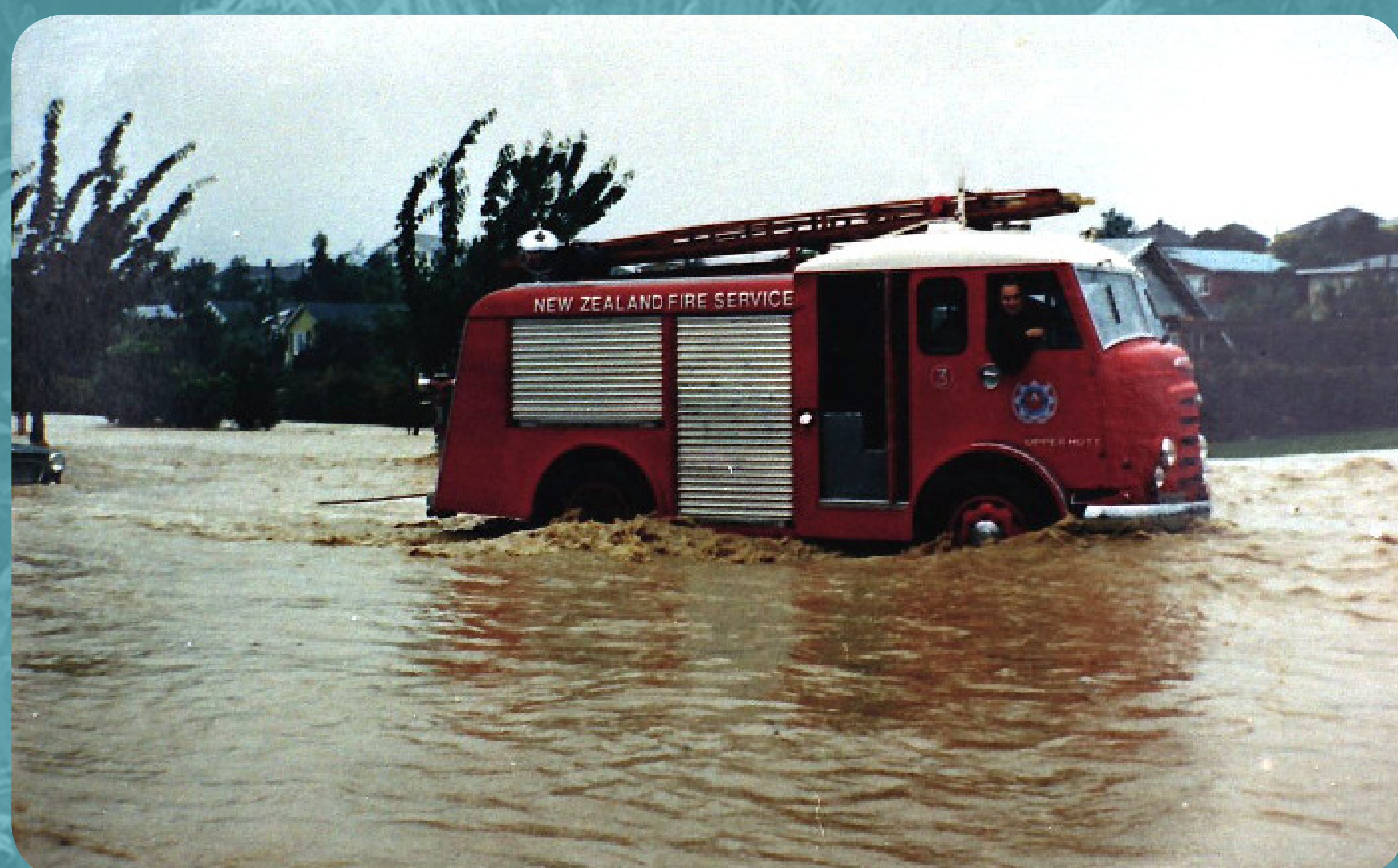
Flooding in the Pinehaven Catchment during the 1976 storm
